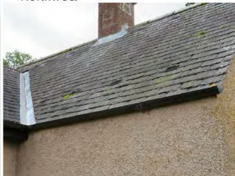
Wall head and chimney
