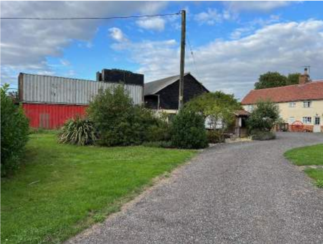
Photo 1. View of existing habitats including shrubs and grassland area 1 within footprint of proposed Scheme. Photograph taken on 23 September 2023.
