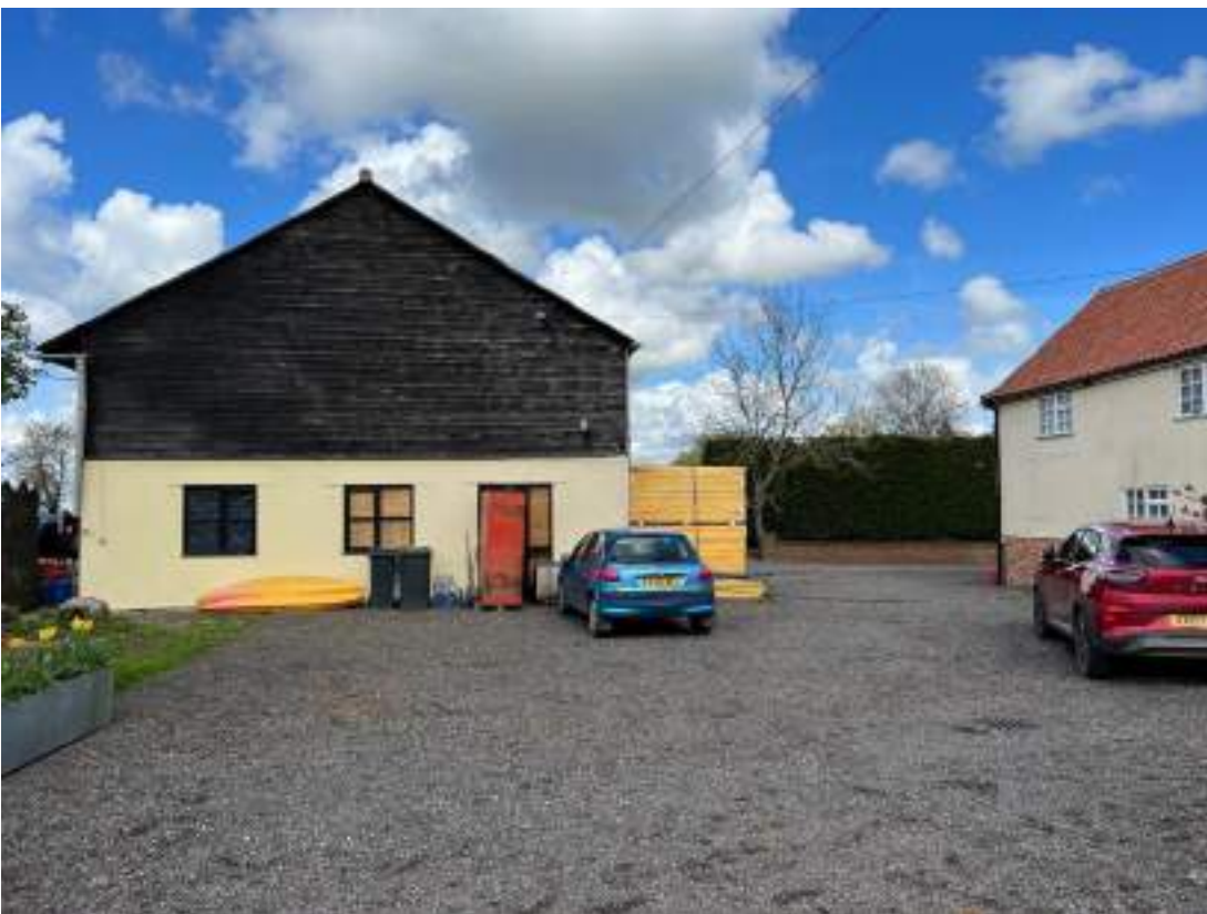
Photo 28. Building 3 to left and Building 5 (Lawn Farm House) to right. Also shows compacted driveway. Photograph taken in spring 2023.
