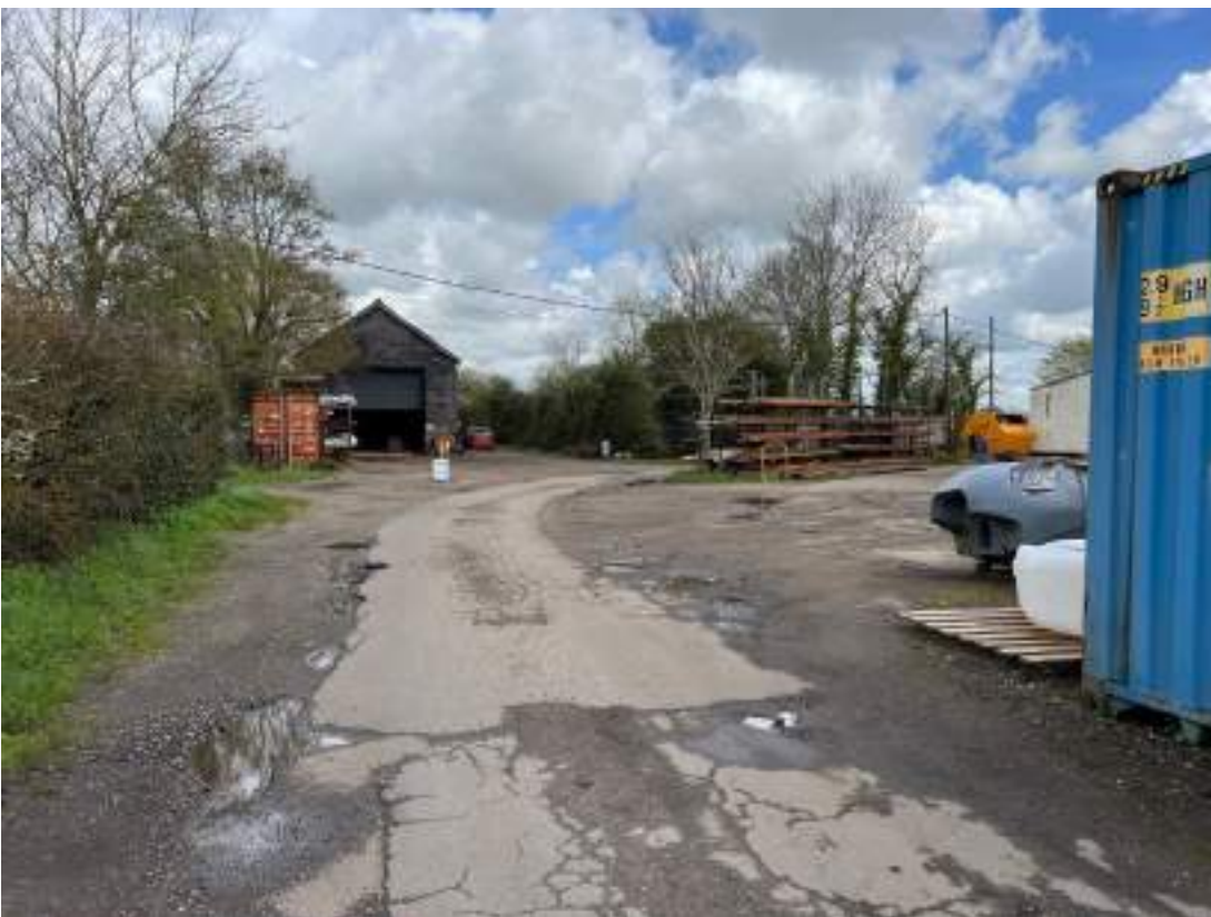
Photo 30. Taken along Metfield Lane. Shows additional ungated access to service yard, common ash tree (T2) and building 4 in the background. Photograph taken in spring 2023.
