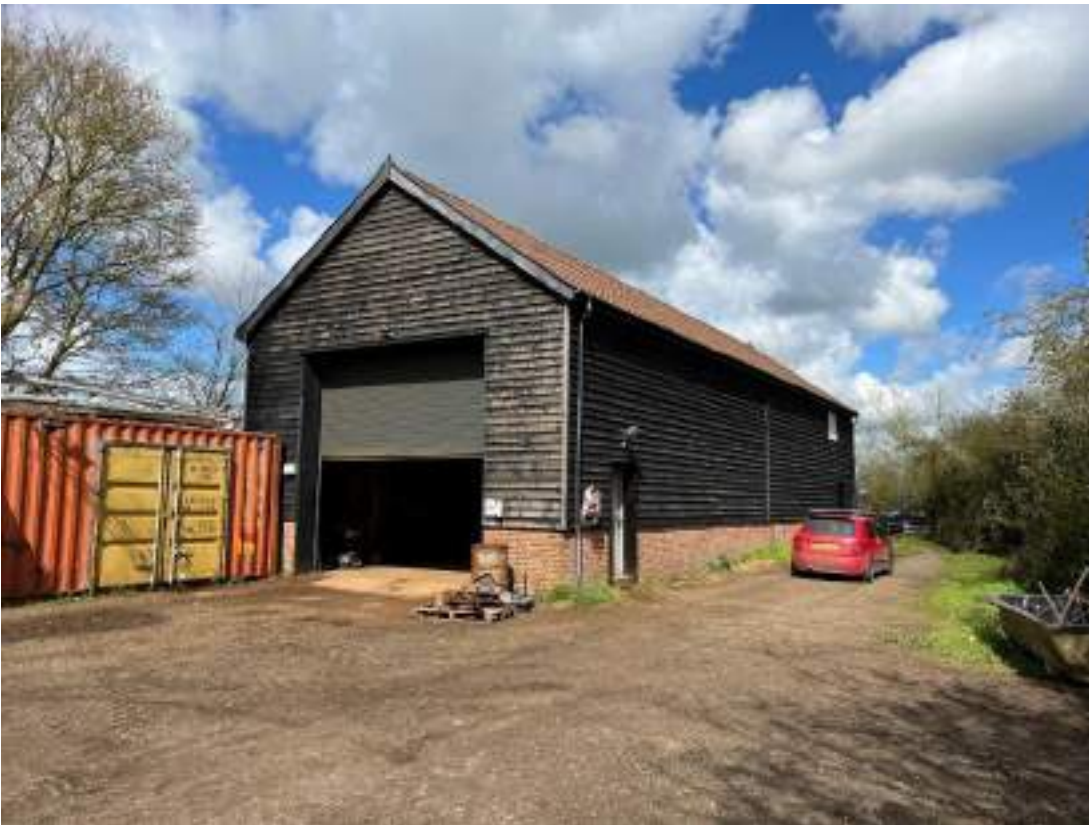
Photo 29. Building 4 along with compacted gravel and ground. Photograph taken in spring 2023.
