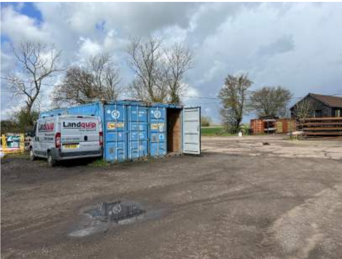
Photo 32. Taken from centre of service area. Shows compacted gravel ground and areas of concrete. Photograph taken in spring 2023.
