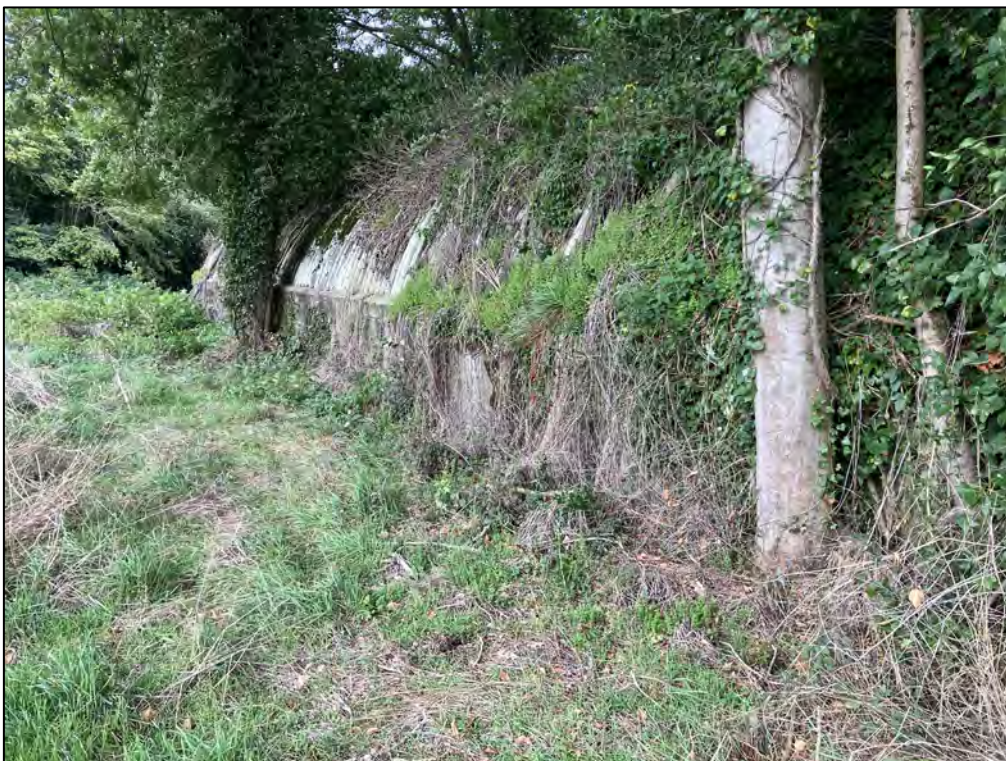
Photograph 8: The barn's southern side, looking towards the west.
