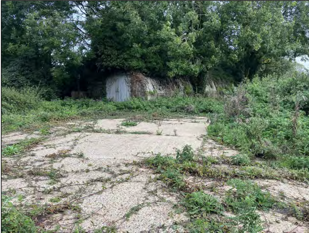
Photograph 5: The hardstanding in the western sector, leading to the barn.
