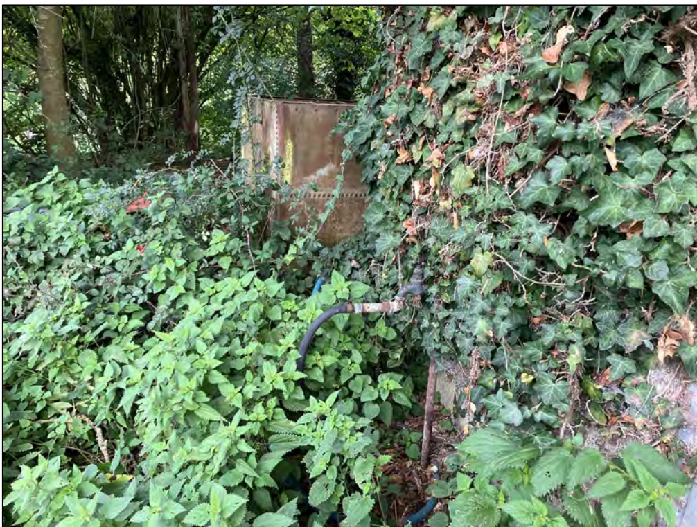
Photograph 6: Water tank adjacent to the barn and tap into the barn.
