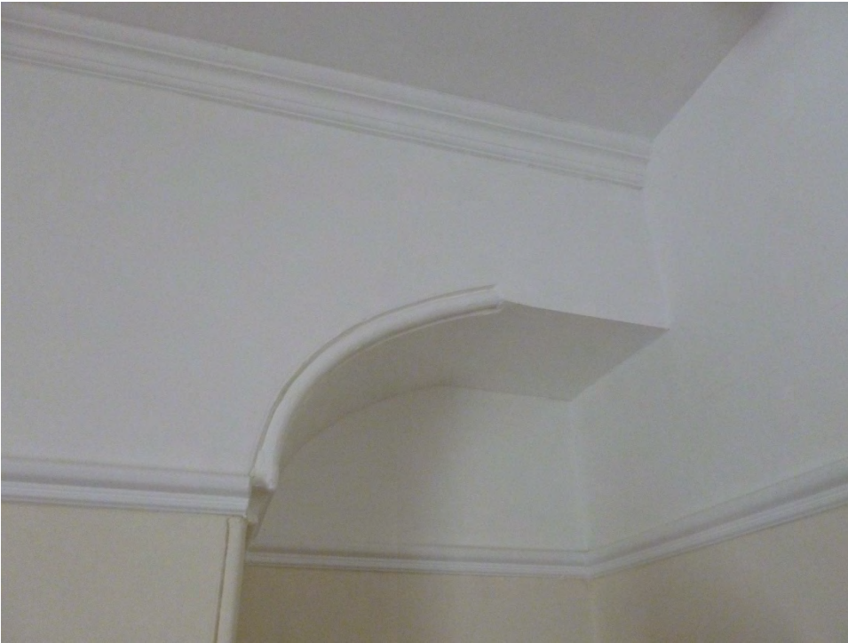
Plate 7: Blocked & divided double door between 'Dining Room' & SW reception Room
