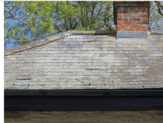
Northeast aspects – missing, lifted tiles and ridge tile gaps.
