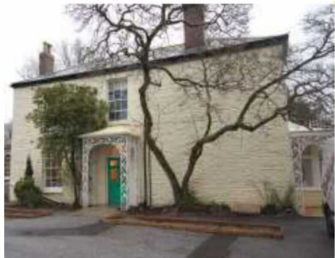
Figure 10 – Principal West Elevation
