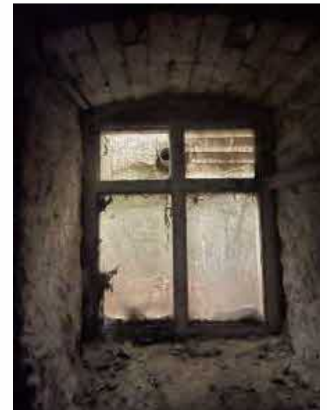
Figure 51 – Photo of basement window
