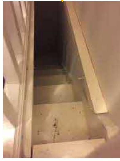
Figure 27 - Original stairs protected
