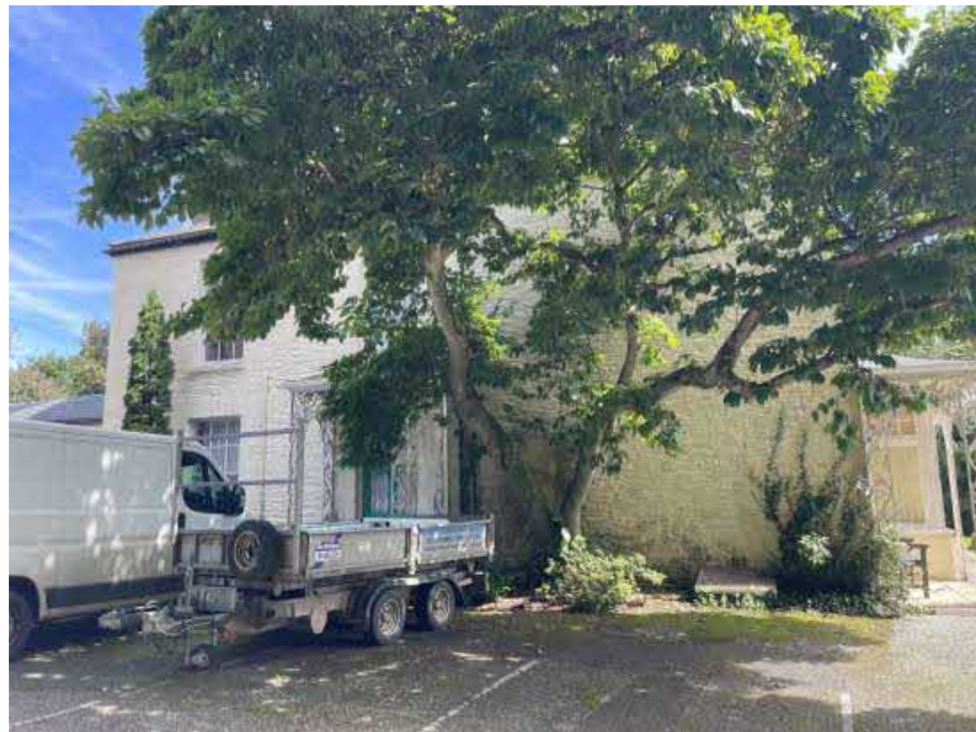
Figure 52 – Photo - South Elevation View of existing lightwell access
