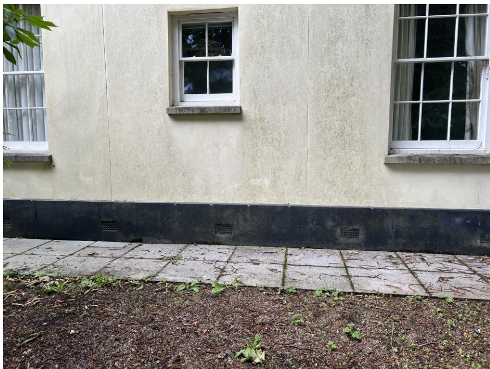
Fig 8 Sub-floor vents in modern extension.
