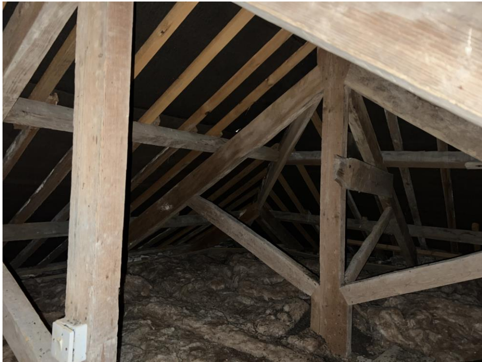
Fig 17 Typical roof structure showing hip end.
