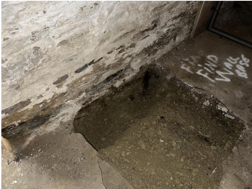
Fig 19 Excavation to underside of basement wall.
