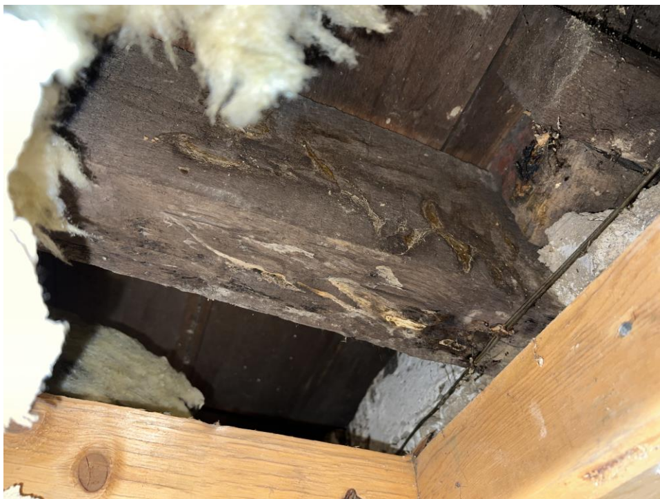
Fig 20 Ground floor joists exposed in basement.
