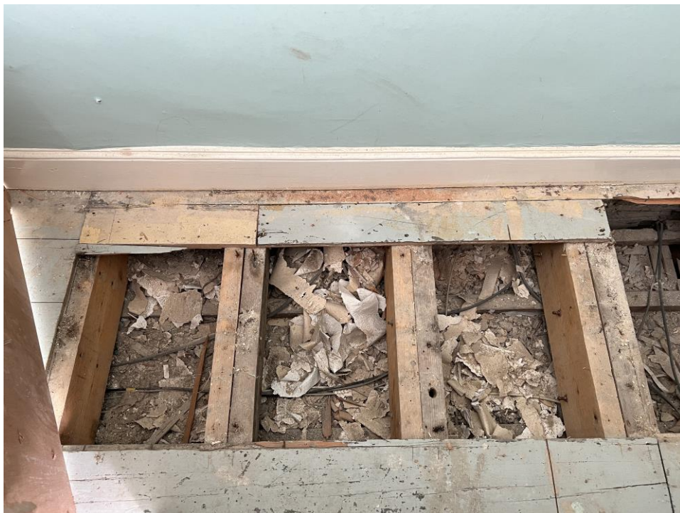
Fig 16 Previously repaired first floor joists.
