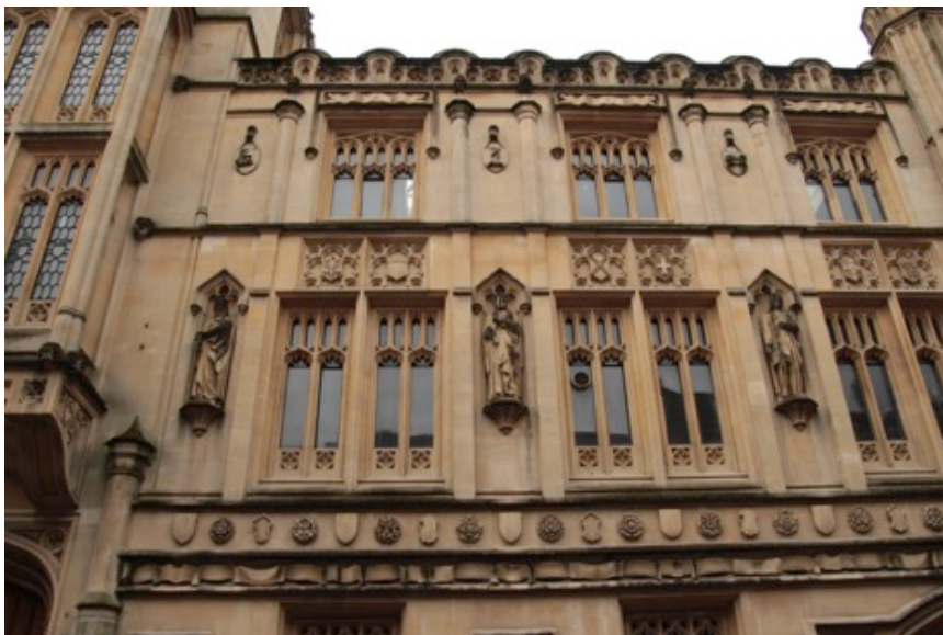
The Broad St facade of Bristol Guildhall showing stone statues by John Thomas
