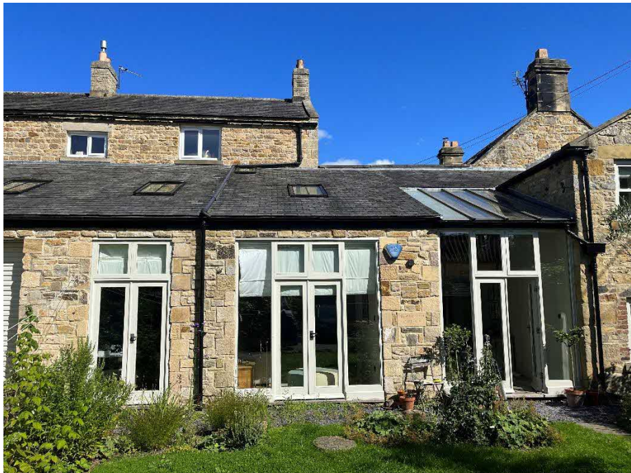
Windows to be reduced in height, new doors and windows to be replaced to match existing system in adjacent opening, see below to note lower head height of adjacent windows/doors.
