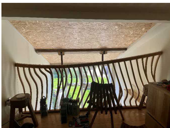
Internal view of glazed roof protection
