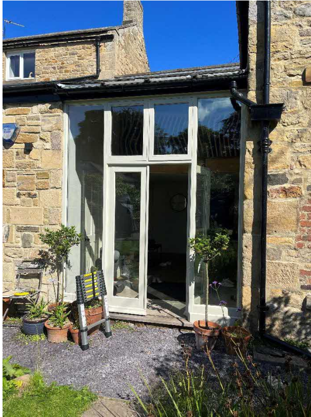
Windows to be reduced in height, new doors and windows to be replaced to match existing system in adjacent opening, see below to note lower head height of adjacent windows/doors.
