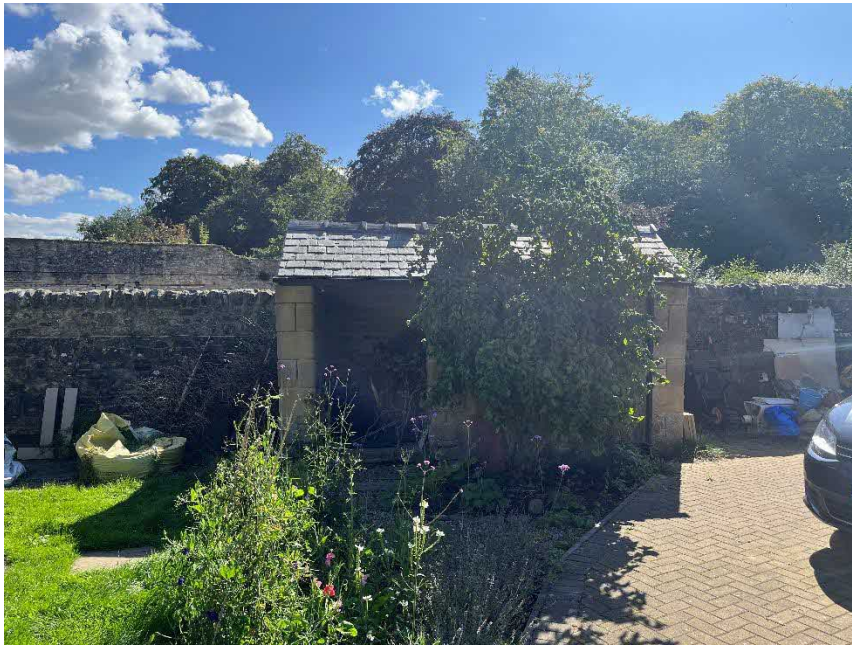
Retained outbuilding, block pavers to be removed
