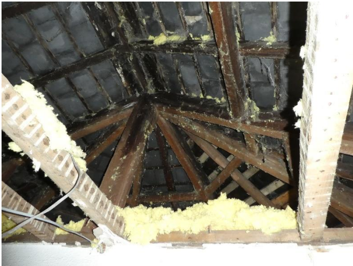
Roof space, Liv Room, looking East and South
