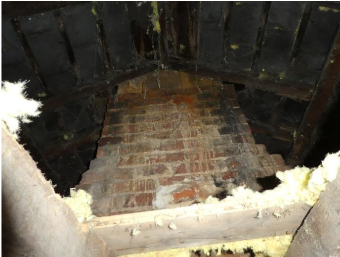
Roof space, Liv Room, looking West, chimney stack
