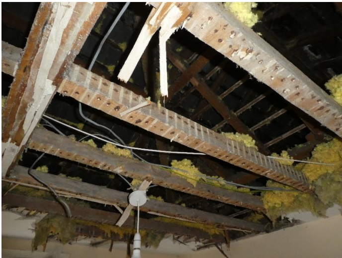
Roof space, Liv Room, looking North West,
