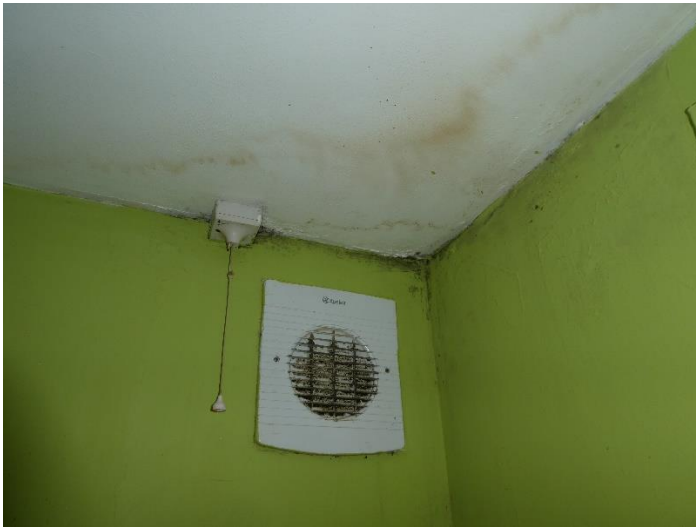
Kitchen North West corner, high level
