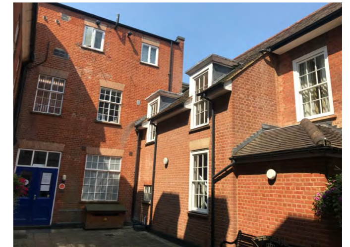
Courtyard view looking North West
