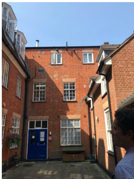
Courtyard view looking West
