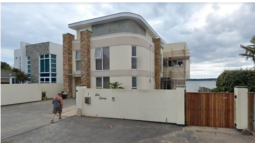
Front Elevation of Sea Spray 1 Gardens Road, Poole. Image source: googlemaps
