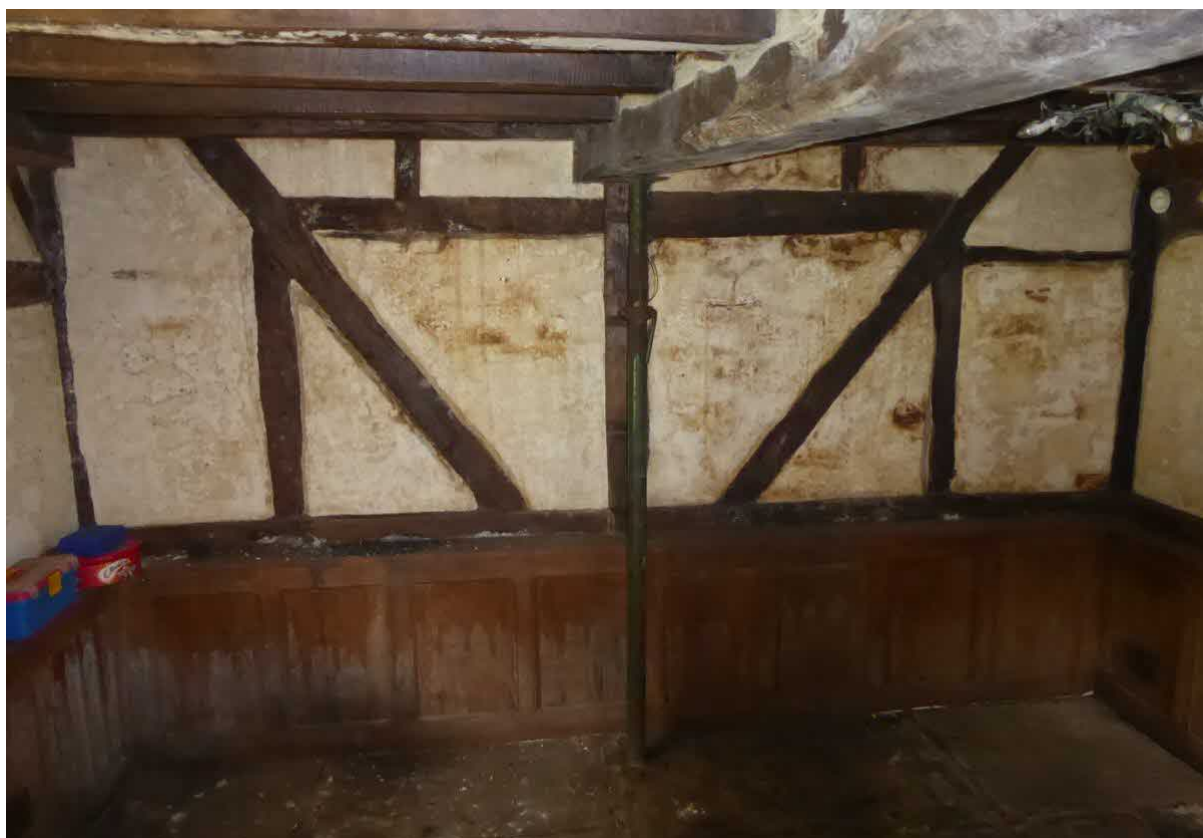
Figure 8: Room G1 – framing to west wall (now internal wall with G3)
