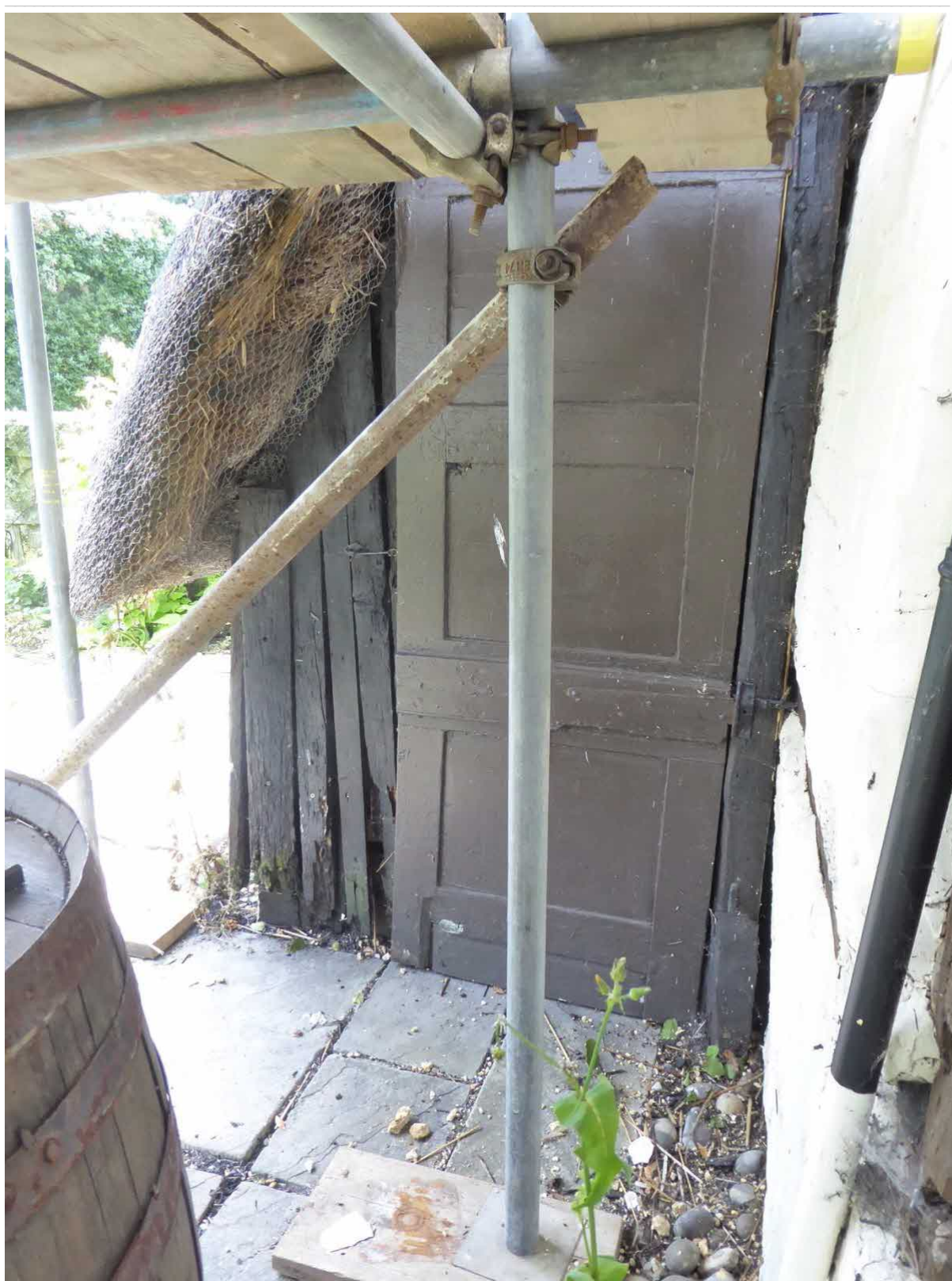
Figure 6: Store to east elevation – north side
