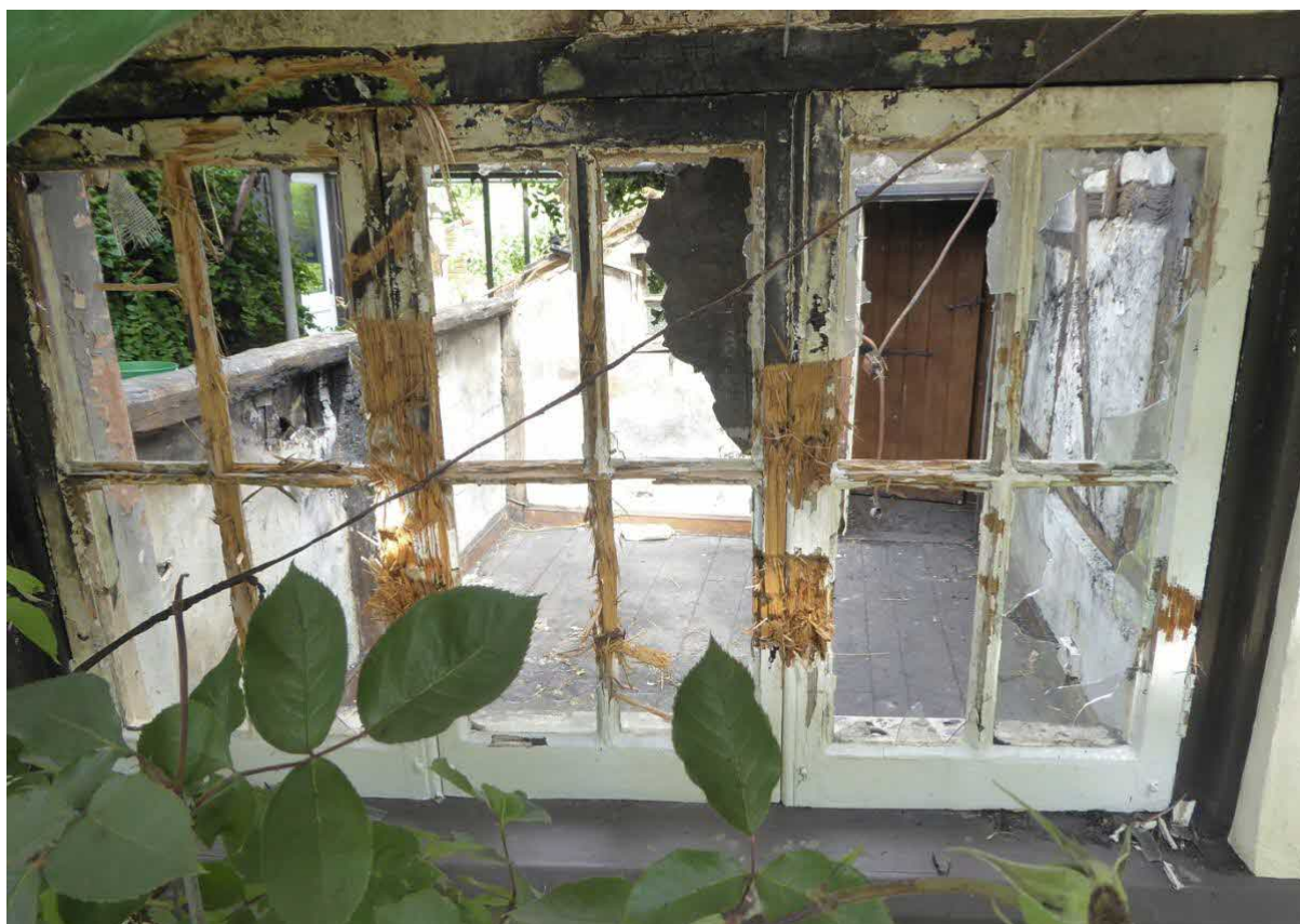
Figure 14: Window W1 (external view)
