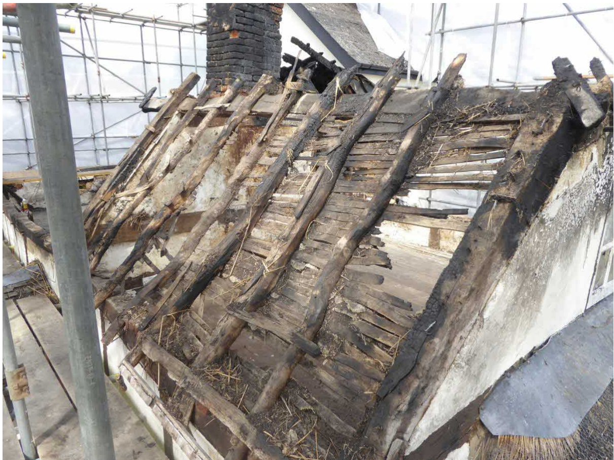
Figure 20: Room F2 -surviving section of roof
