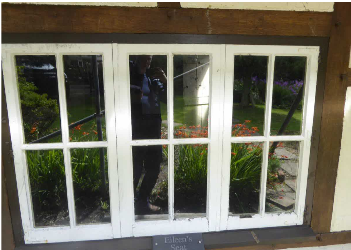
Figure 2: Window W2 – part of c2000 restoration works
