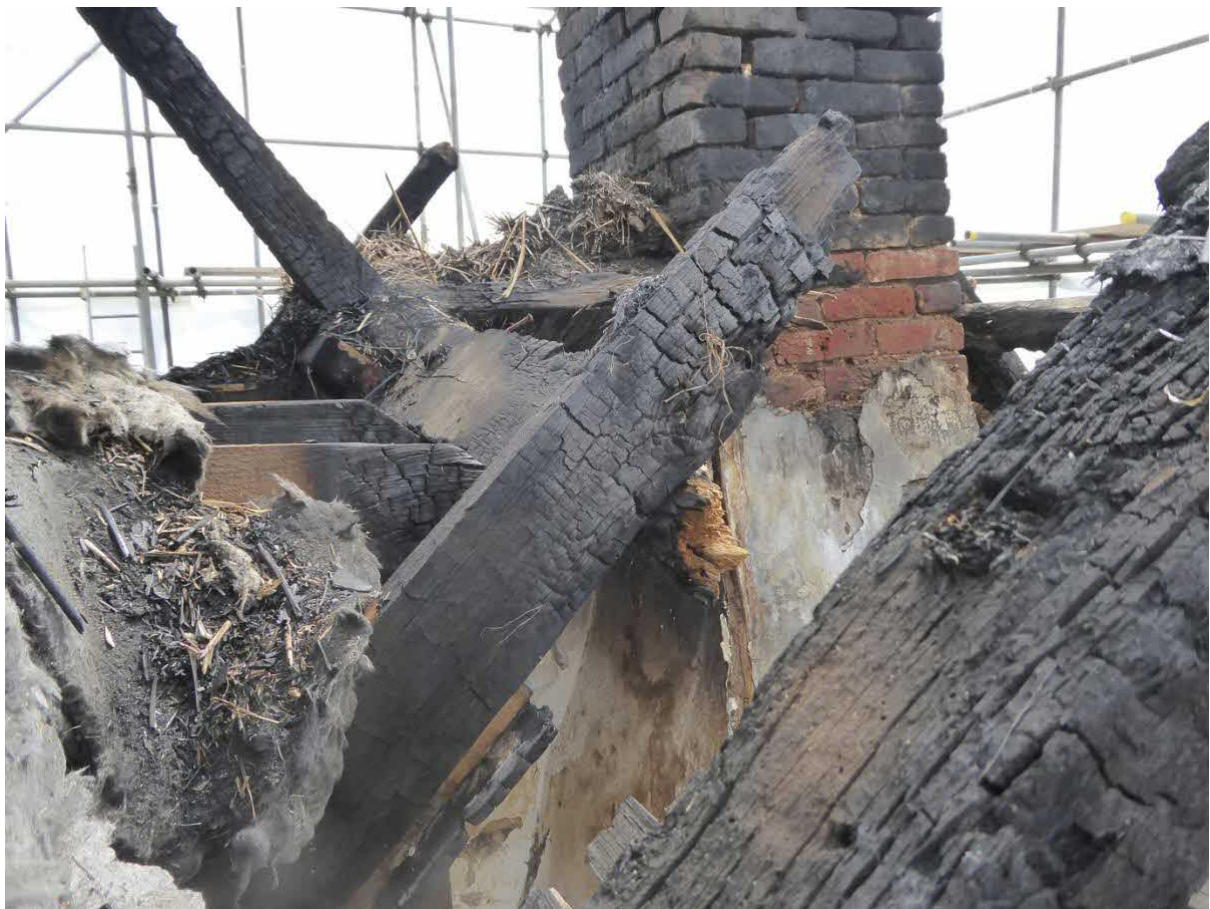
Figure 18: Small section of roof above landing/stair
