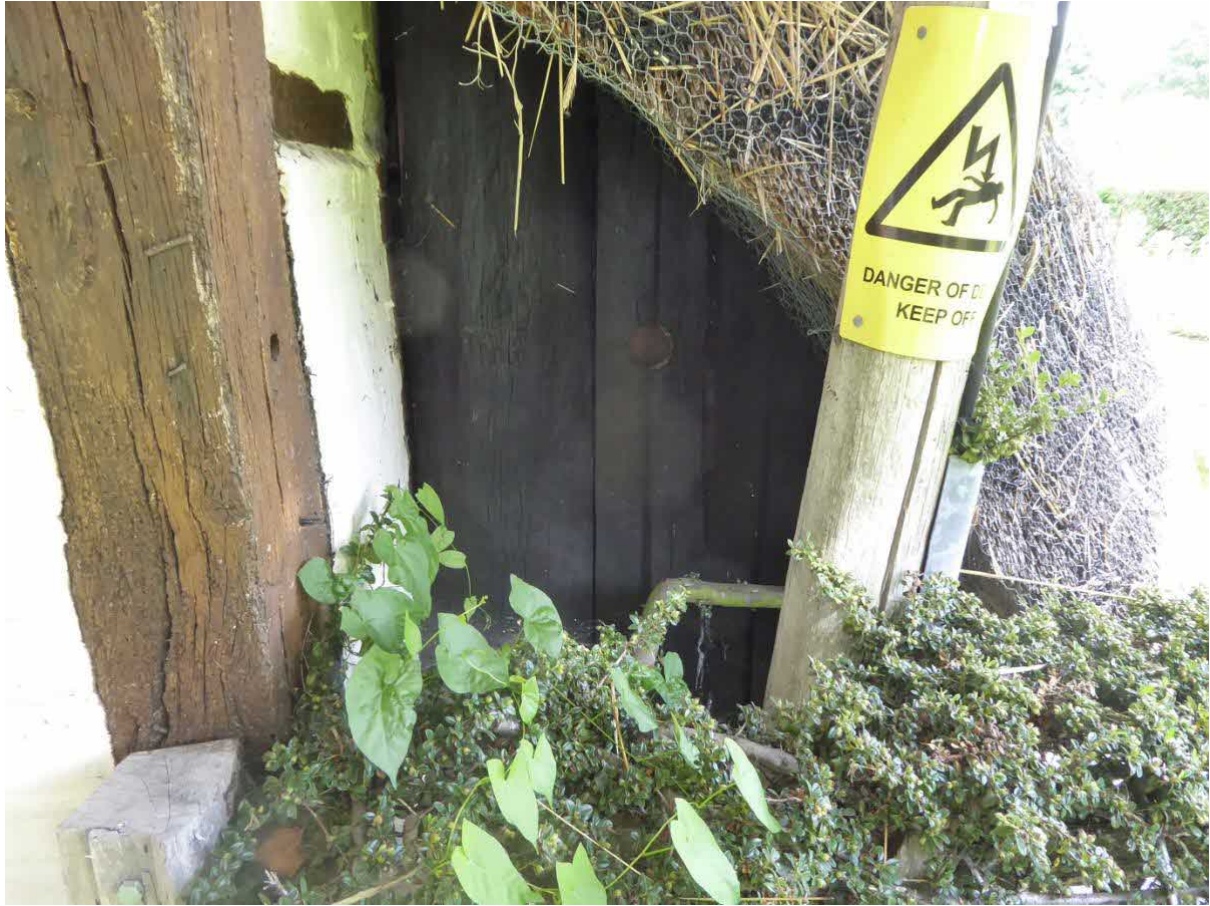
Figure 5: Store to east elevation -south side
