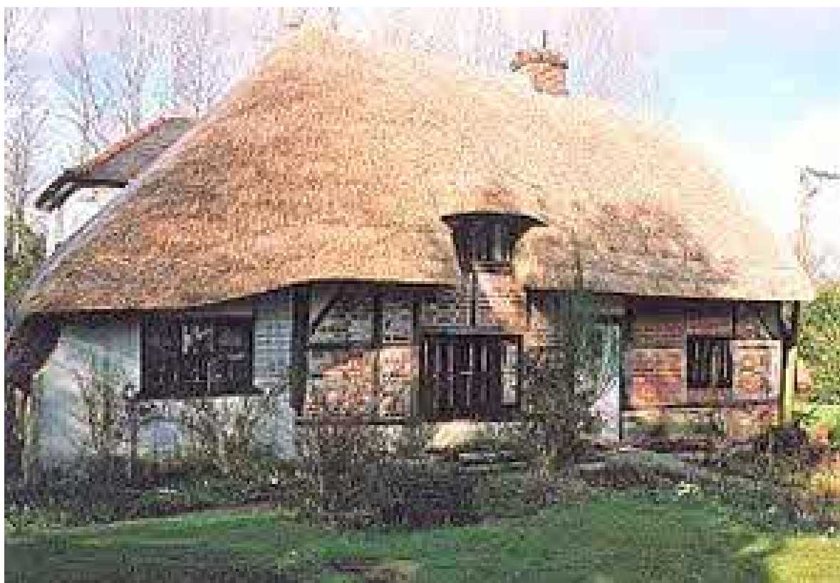
Figure HP4: Wellow Wood Cottage – post c2000 restoration and post-rethatching
