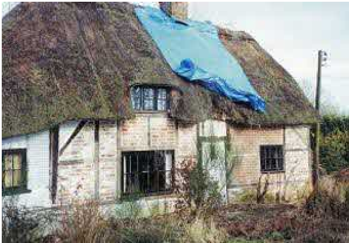
Figure HP1: Wellow Wood Cottage – post c2000 restoration (pre-rethatching)
