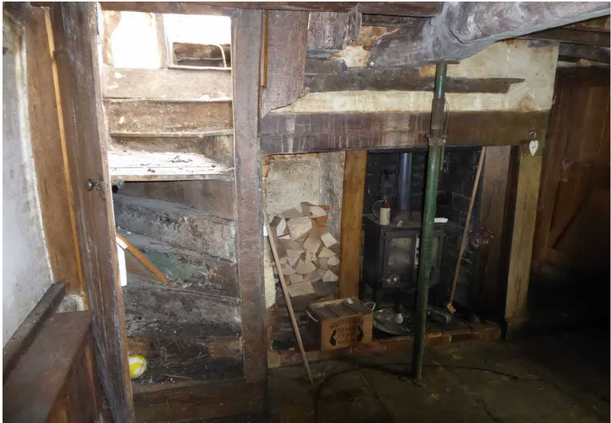
Figure 9: Room G1 – fireplace and staircase (floored at first floor)
