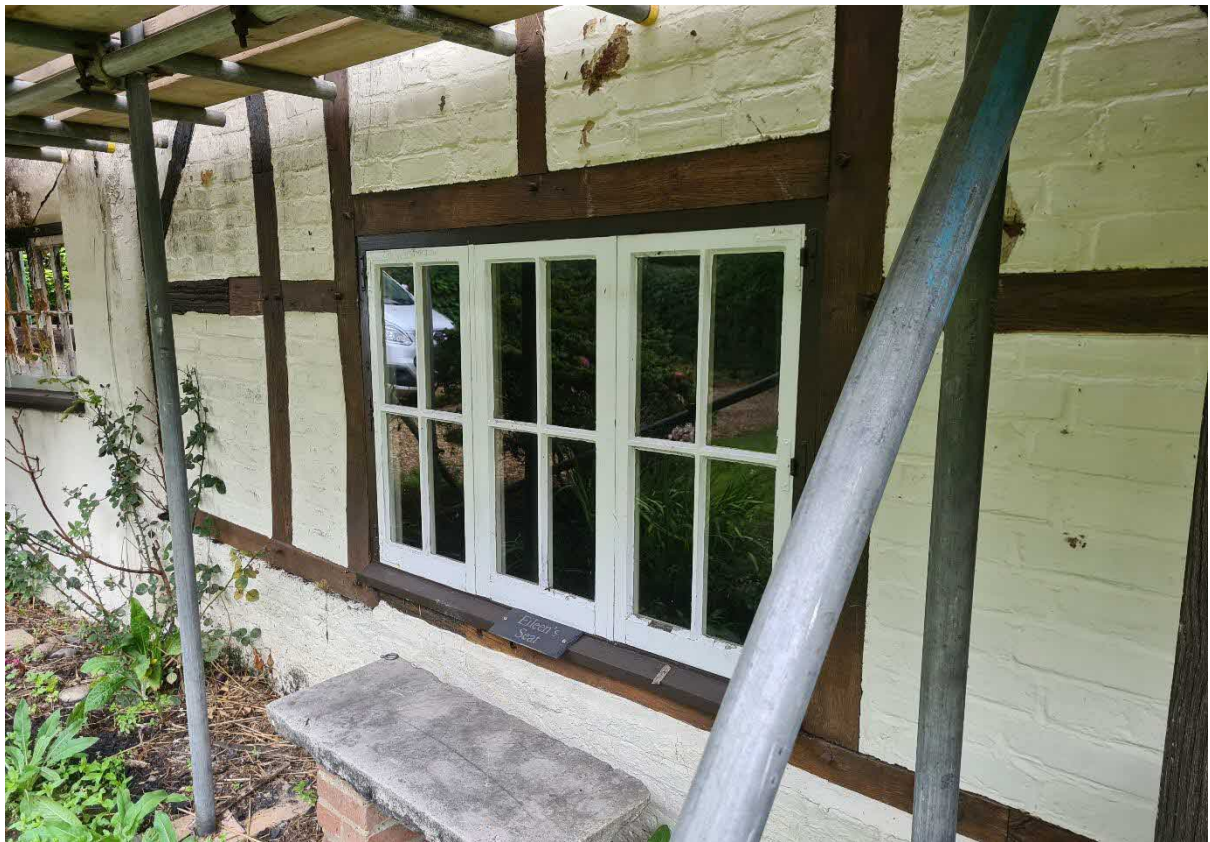
Exterior view at southwest corner of frame. This area of framing has been rebuilt to a good standard, although historically there would have been a jowled storey post in the middle of the window. I suspect that the current window replaces a Victorian window which cut through the post making restoration of the post seem pointless to previous occupants.
