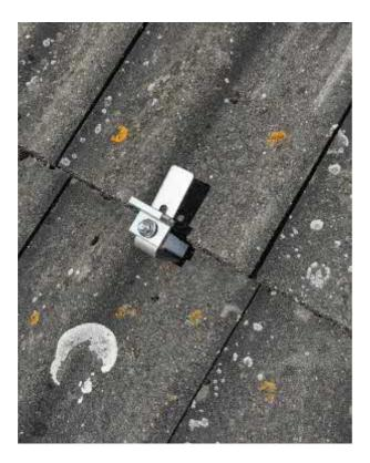
4. A further example below. As you can see the bracket includes the "seat" for the rail so that 39mm rail thickness is included into the brackets profile as per the dimensions shown above.
