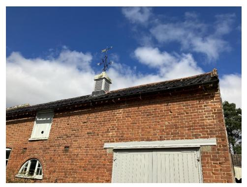
Photograph 7 – Previous repairs to Coach House South Elevation. Minor distortion of brickwork bed joints over double door opening.
