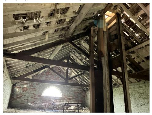
Photograph 12 – Timber roof structure to Coach House.
