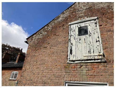
Photograph 5 – Coach House East Elevation. Efflorescence of brickwork at high level and localised spalling of brickwork.
