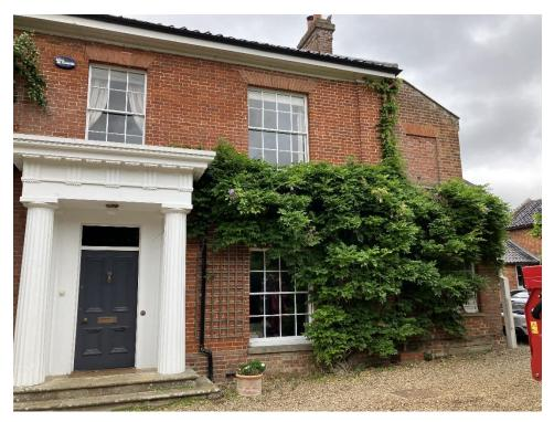
Photograph 4 – Main House Lean-to East Elevation. Efflorescence of brickwork at high level and brickwork repairs under ground floor window. Historic window opening infilled at first floor.
