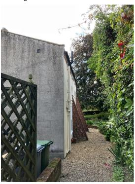
Photograph 2 – View of buttresses to Main House West elevation. Minor staining of brickwork at base of buttresses.
