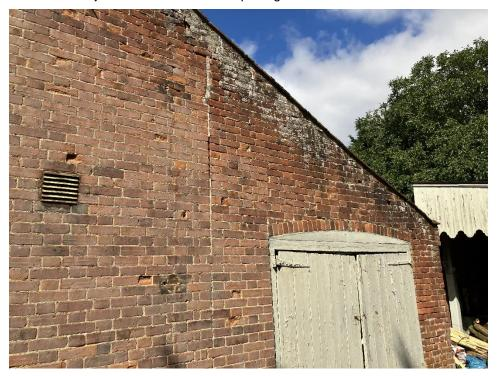
Photograph 8 – Vertical joint in Coach House East Elevation.
