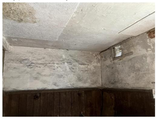
Photograph 10 – Cracking in corner of stable area. Crack extends through the wall and is visible in the adjacent garage.
