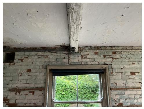
Photograph 11 – Diagonal cracking over brickwork over Coach House garage window opening. It appears that no lintel has been provided above the window.
