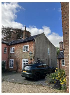
Photograph 3 - East Elevation of Main House Service Wing. Staining of brickwork between ground / first floor windows and previous repairs to brickwork. Localised spanned bricks.
