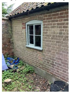
Photograph 14 – Cracking and previous brickwork repairs to Garage rear elevation.
