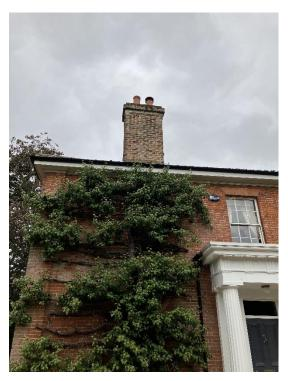
Photograph 1 – View of chimney adjacent to Southeast corner of Main House. Efflorescence / staining of brickwork visible on brickwork behind tree.
