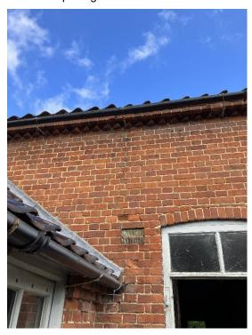
Photograph 6 – Vertical crack on Coach House South Elevation.
