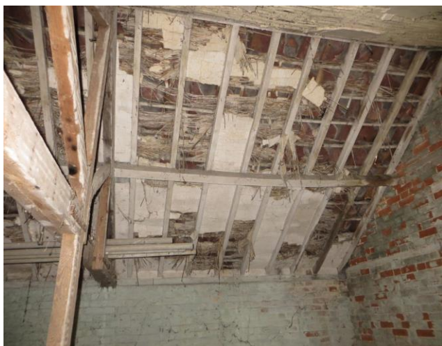
Roof area of Coach House inside main area.
