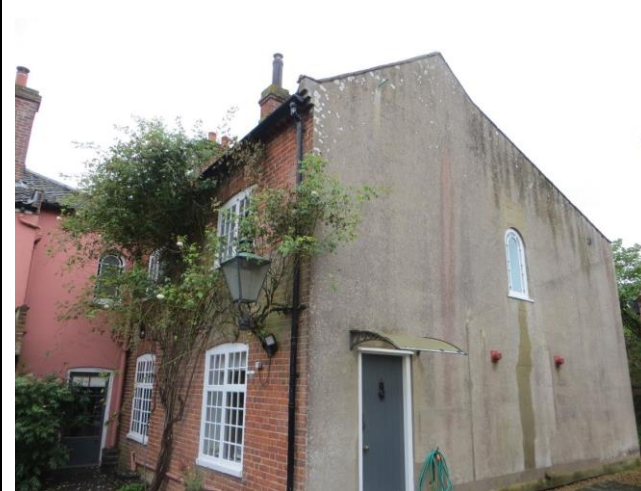
Service wing. Northern (rendered) and eastern (brick) elevations.
