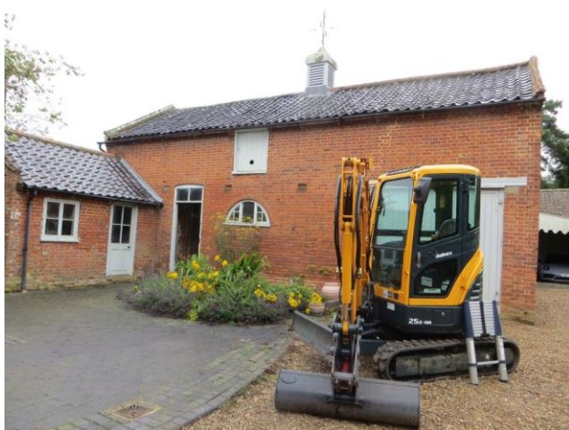
Southern elevation of Coach House and Coal Store to the left of photograph. Photographer facing north.
