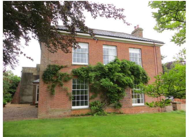
Southern elevation of Fern House.
