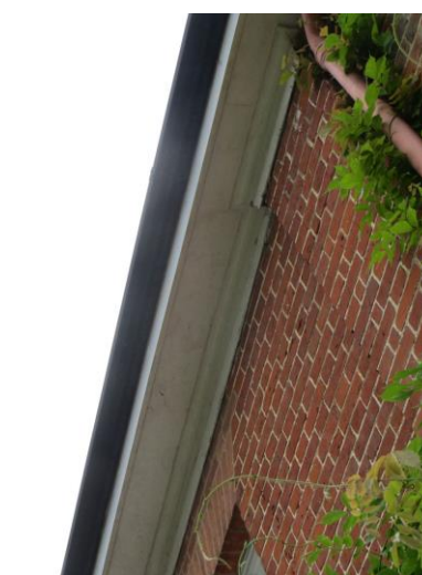
Sealed soffit box.
