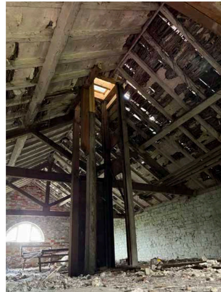
Photo from inside stable/coach house roof space
