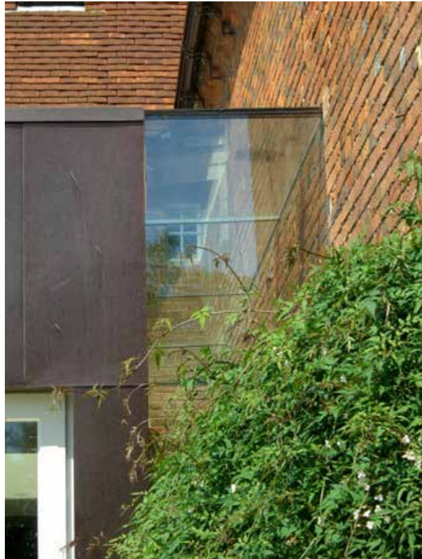
Precedent image; Hudson Architects utilised glazed abutments at grade II listed Quaker's Hall in Broadland to express the separation between new and old.
