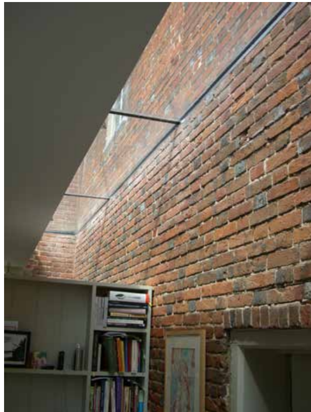
Precedent image; Hudson Architects utilised glazed abutments at grade II listed Quaker's Hall in Broadland to express the separation between new and old.
