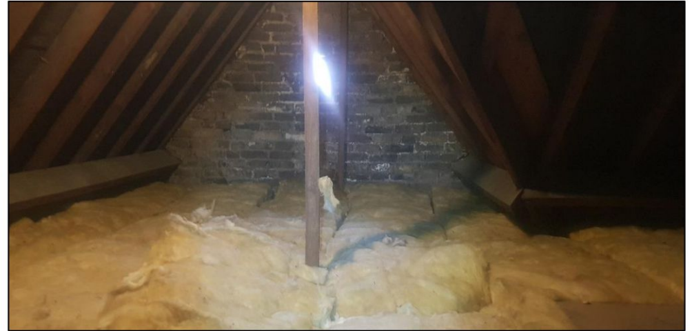
Picture 3: Inside loft space of B1 looking south
