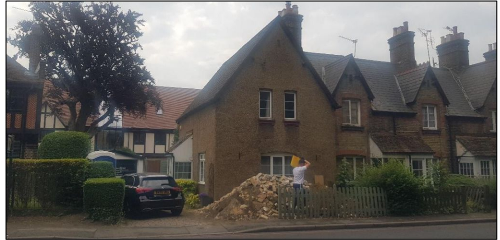
Picture 1: Looking south-west at the northern and eastern elevations of B1
