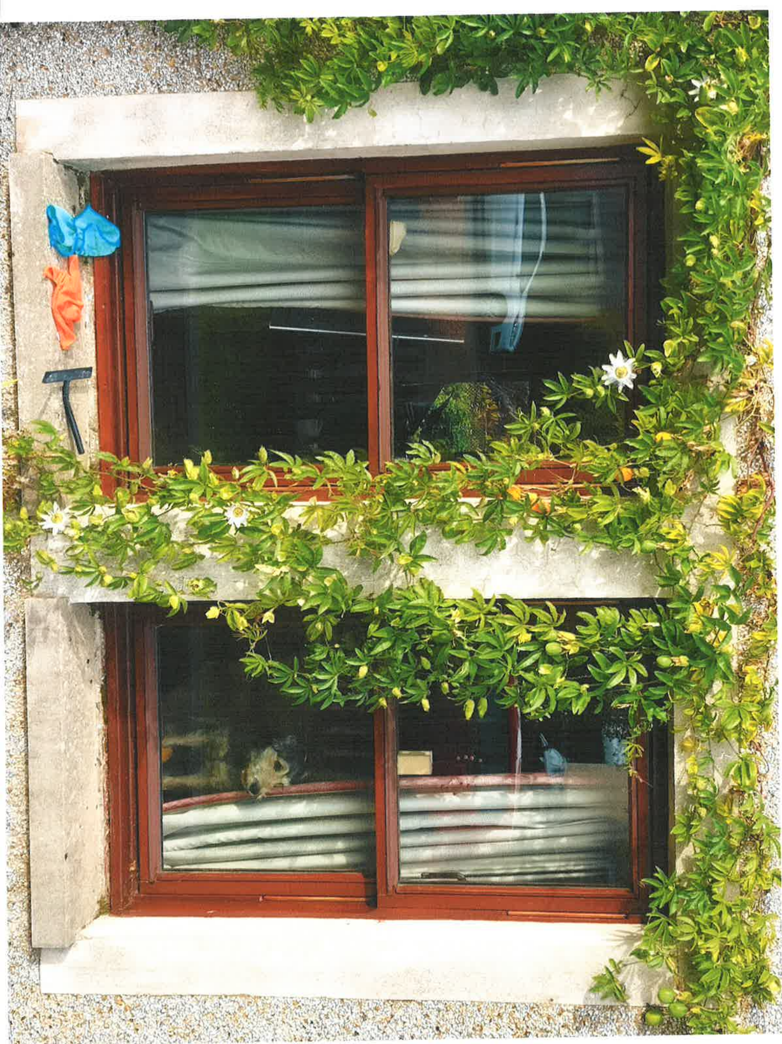
EXISTING FRONT GROUND WINDOWS
