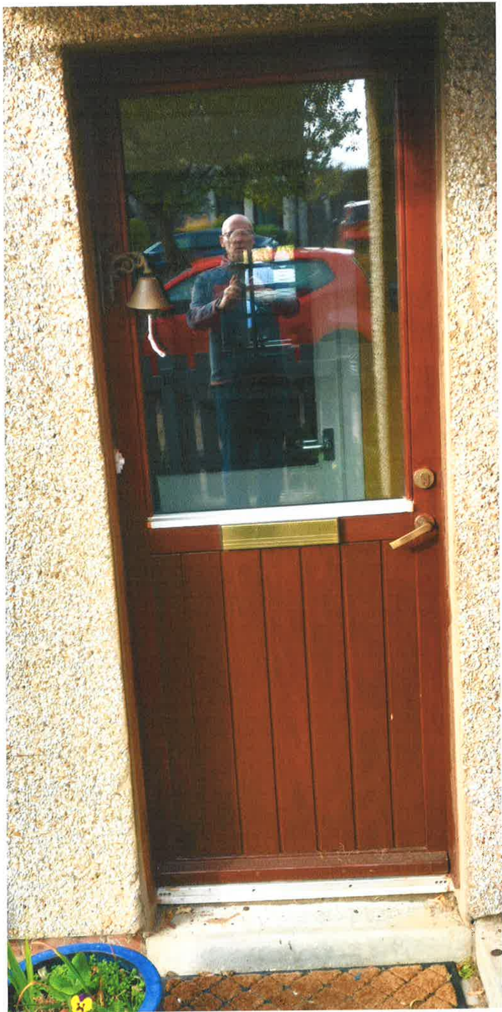
EXISTING DOOR (FRONT)
