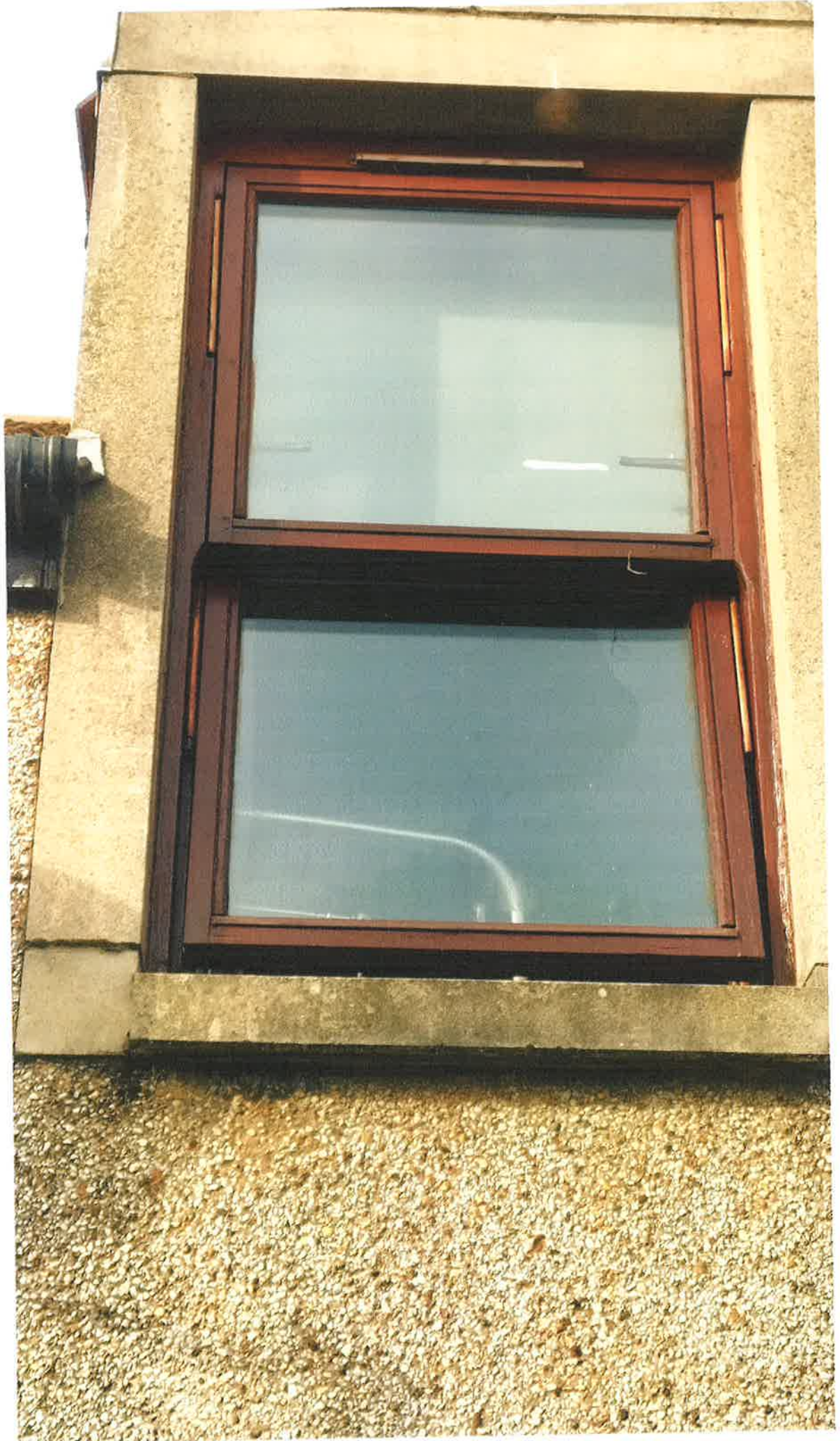
EXISTING FIRST FLOOR FRONT
