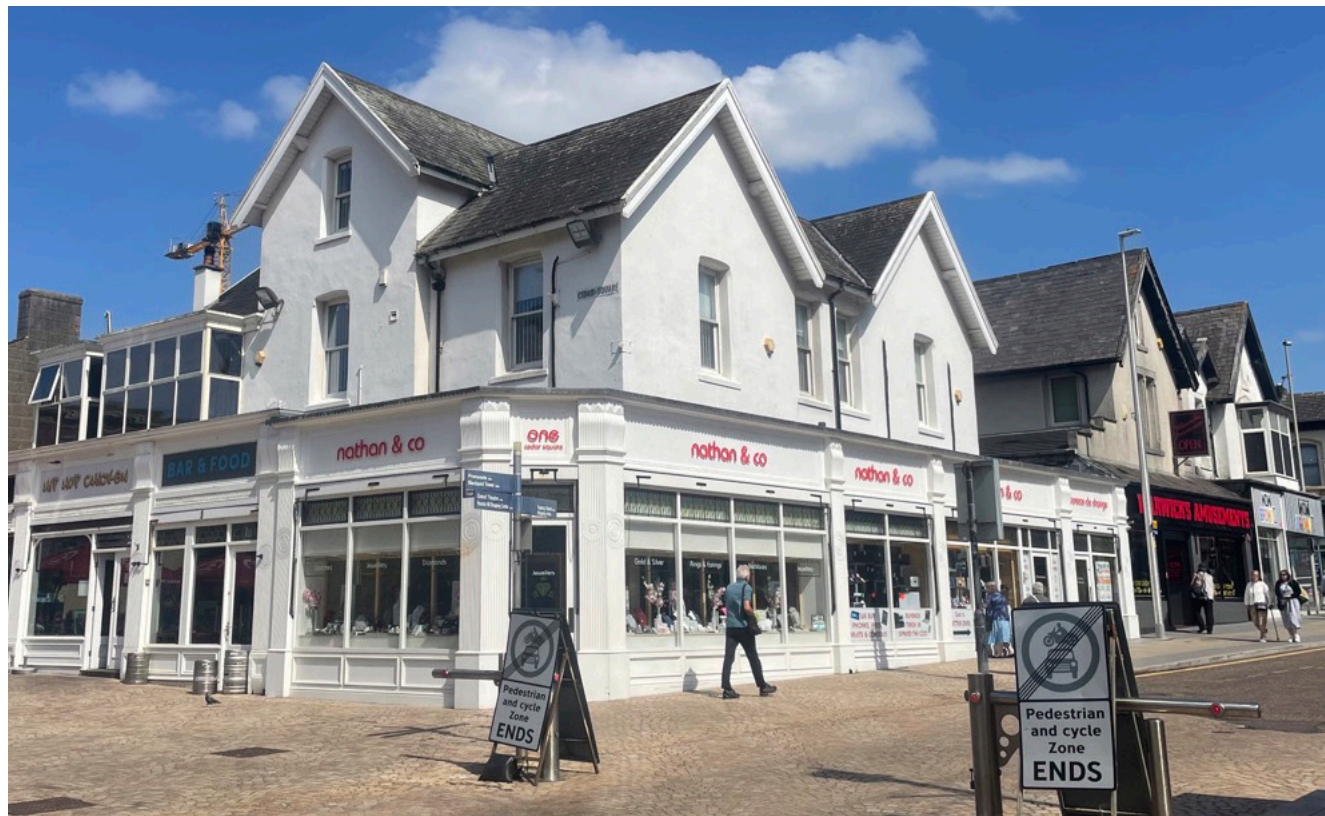
Previous projects undertaken by Joseph Boniface Architects Ltd for the Quality Corridors scheme
