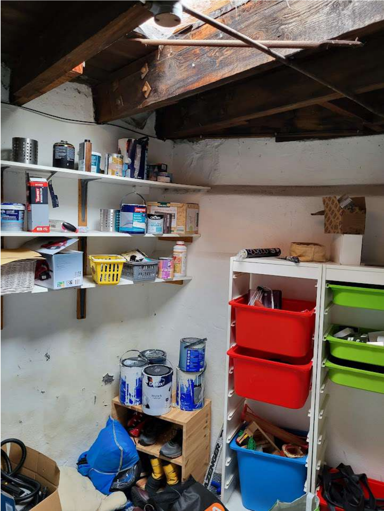
THE EXISTING STORE ROOM TO BE CONVERTED INTO A SHOWER ROOM
