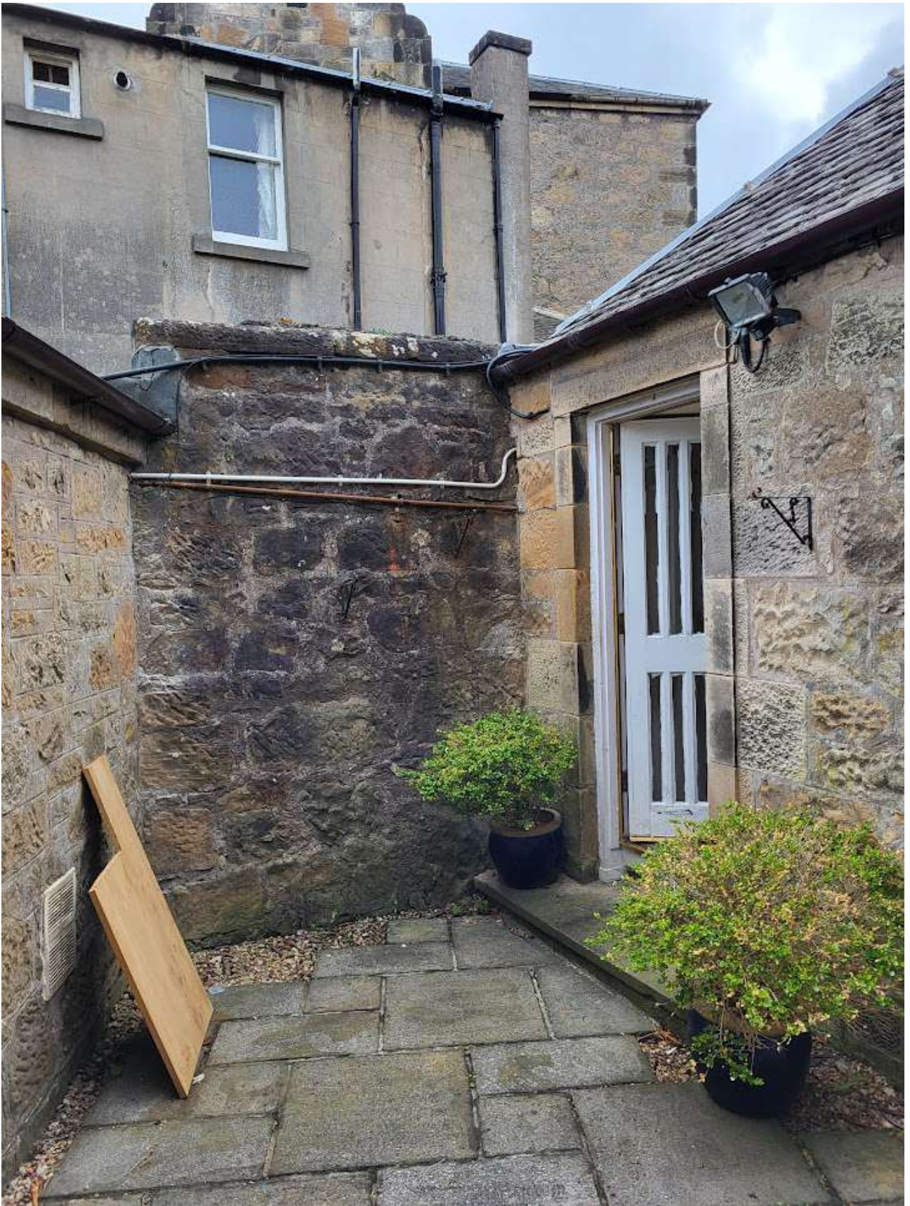
PHOTO OF THE DOOR IN THE COURTYARD TO THE EXISTING OFFICE/STUDIO
