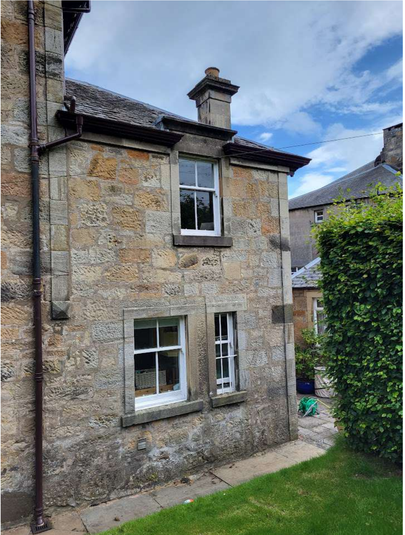
PHOTO OF THE EXISTING UTILITY WINDOW FROM THE OUTSIDE
