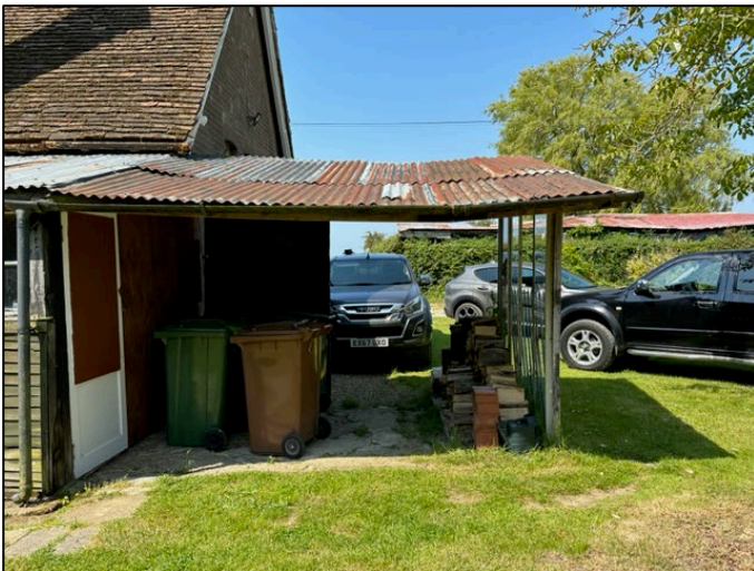
b) Car port and maintained lawn to the north.
