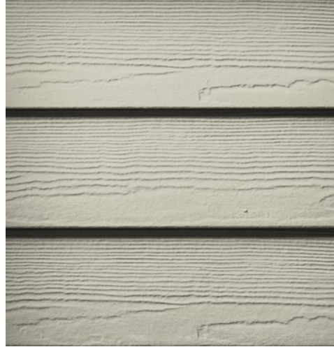
Cladding: Hardi Plank Cobblestone
