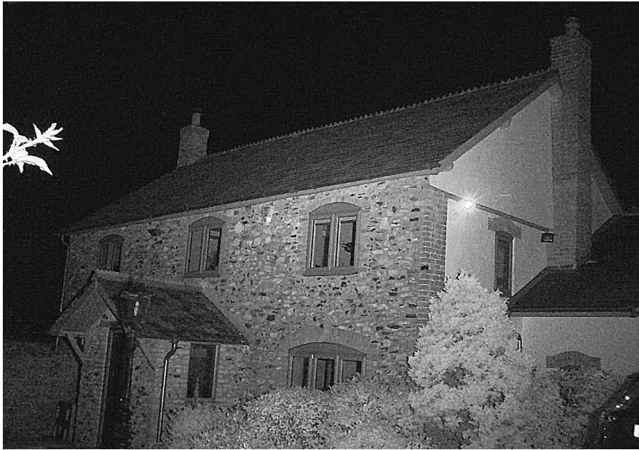
Plate 18 - Eastern elevation - survey 2
