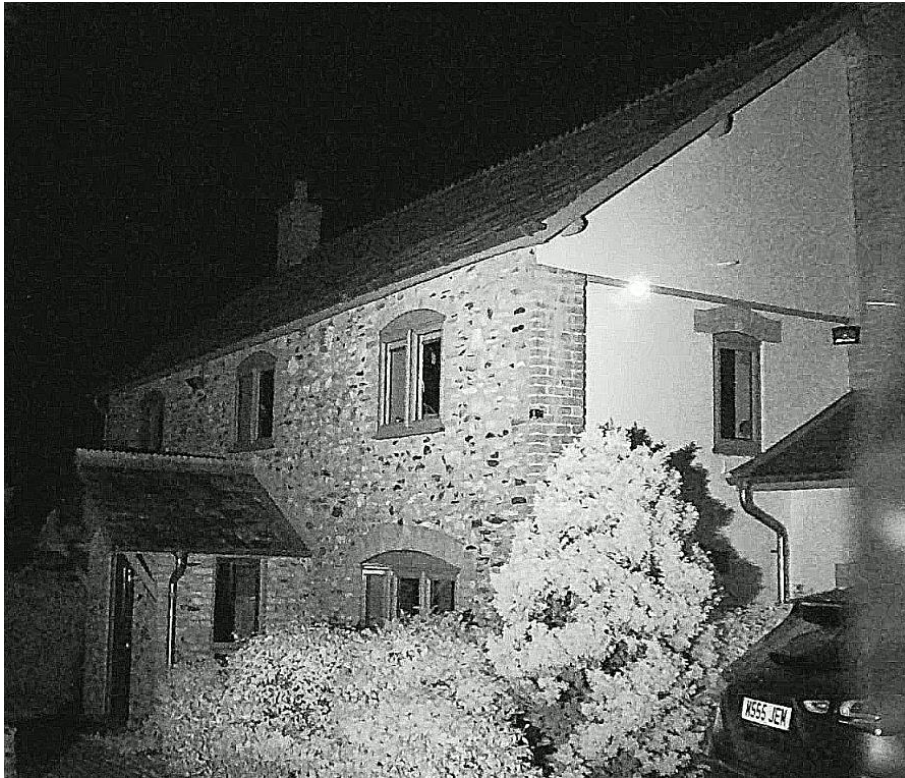
Plate 16 - Eastern elevation - survey 1
