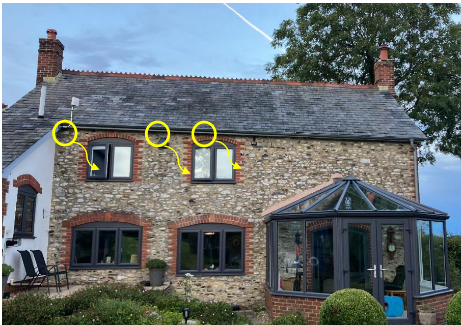
Plate 12 - Emergence/re-entry locations of brown long-eared bats on the western elevation of the house
