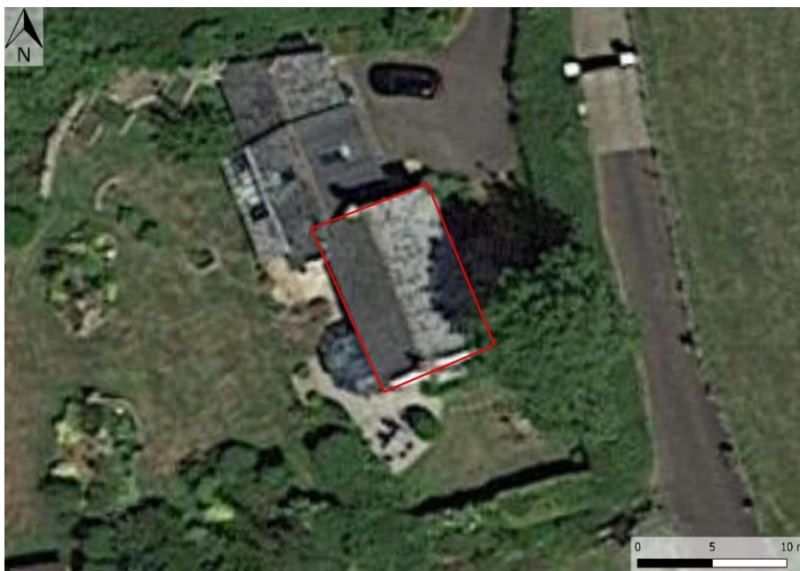
Plate 2 - Close-up aerial photograph showing the site and the building surveyed
