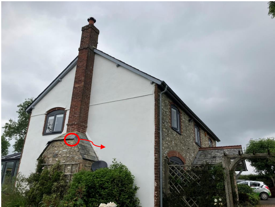
Plate 14 - Emergence location of three common pipistrelle bats on the southern elevation
