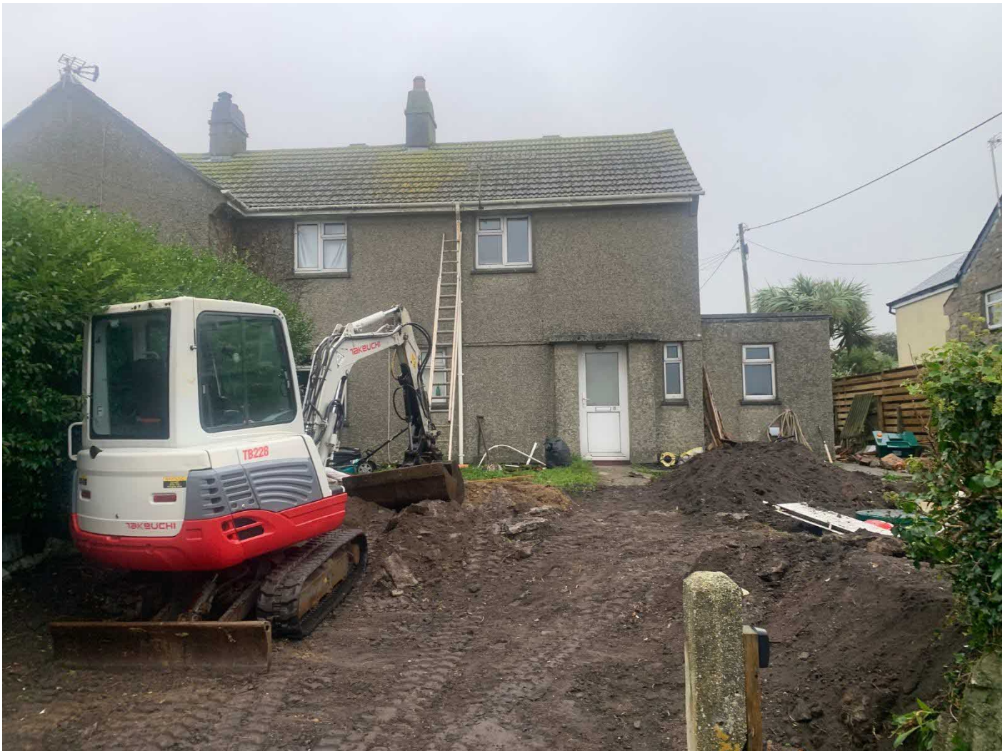
Figure 1: Eastern elevation of property assessed
