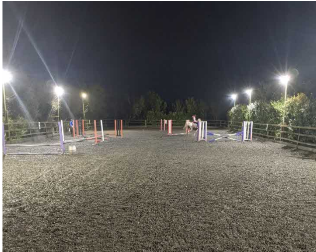
Figure 5: Photo of the existing Flood Lighting at the Sand School
