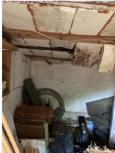
Internal view of outbuildings showing general storage from Woodnook farm
