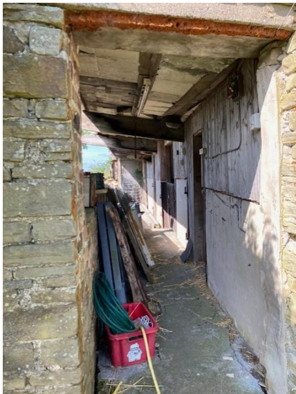
Photo showing existing stone outbuilding with concrete hardstand
