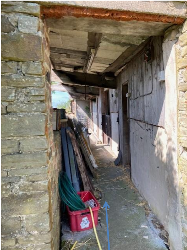
Main structure is stone with block infill on concrete plinth pad (raised)
