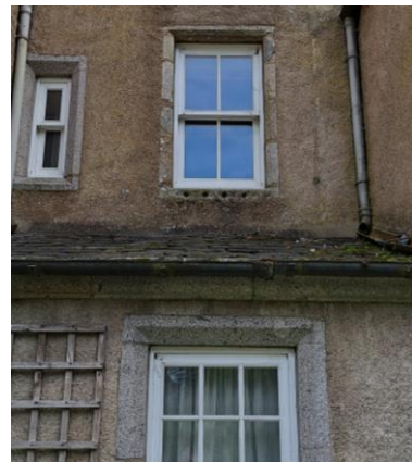
West Elevation Windows Note reused cill on upper window and different chamfer profiles.
