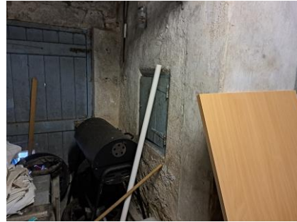
Coal cellar access in garage structure.
