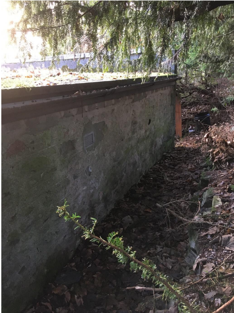
Rear (north) elevation is partially hidden, acting as a retaining wall to the adjacent ground
