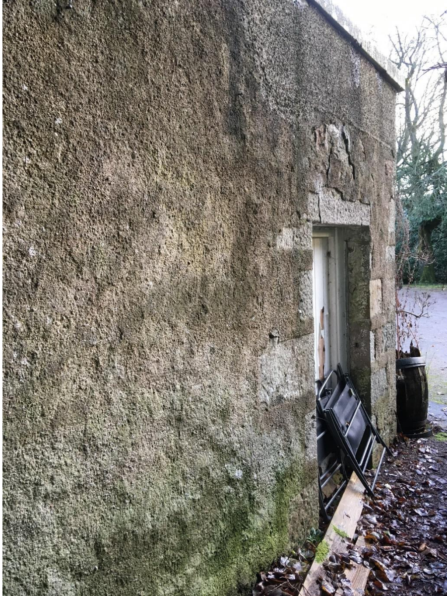
Left hand (west) elevation which has been covered in cement harling
