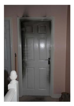
Non fire rated door and 4mm float glass remaining intact, even when fire burnt through the roof
