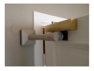
The mechanism should be fitted so that the release button is easily reached, or provided with a remote release button.
