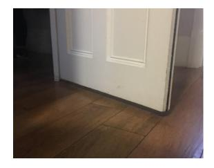
Diagram 5 Gap beneath door caused by sloping floor
