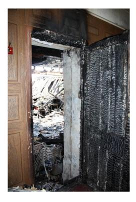
Although older doors and frames were not designed for fire protection, there are some cases where only minor modifications, as shown on pages 14-18 are required, particularly to panel doors to provide 20 or 30 minutes fire resistance in a fire test.
