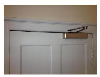
Lipping the top of the door or frame puts the repair in the most critical part of the door set during a fire. If the door can be raised by adjusting the hinges, the lipping can be applied to the bottom of the door.
