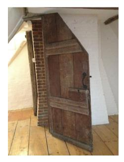
Ledged and ledged and braced doors are susceptible to warping from environmental changes and often have adjusted stops to accommodate the twist of the door.
