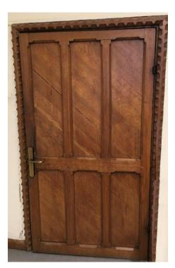
Four panel door provided good protection from a severe fire
