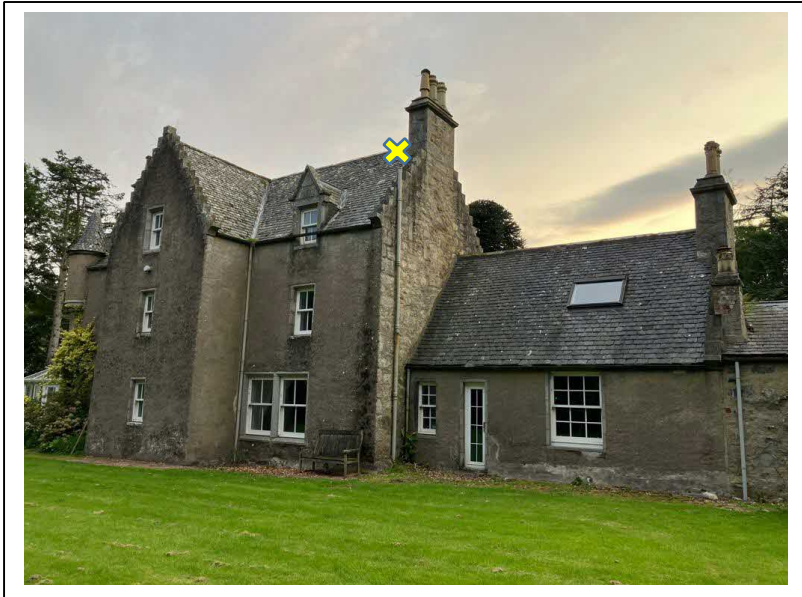
Thermal imaging view west elevation
