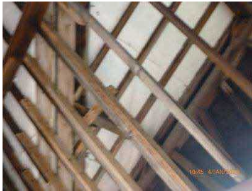
Figure 15. Internal timber roof structure.
