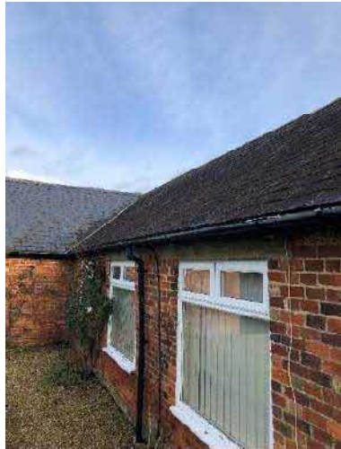
Figure 9. PVC window frames and concrete lintels.
