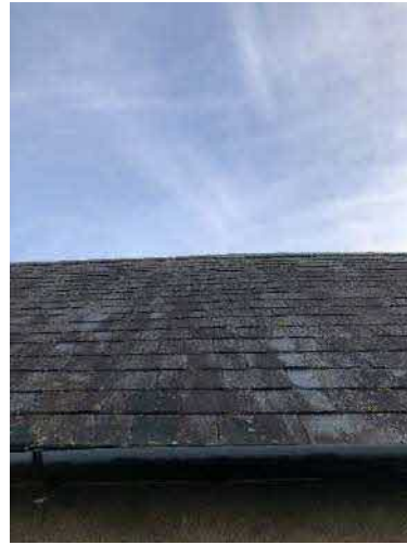
Figure 18. Slate-tiled roof in good condition.
