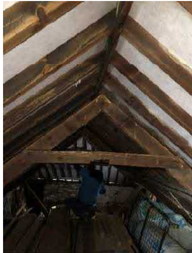
Figure 21. Western roof void.
