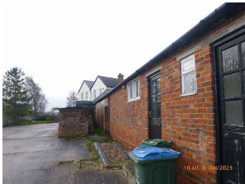
Figure 7. Calf pens building.
