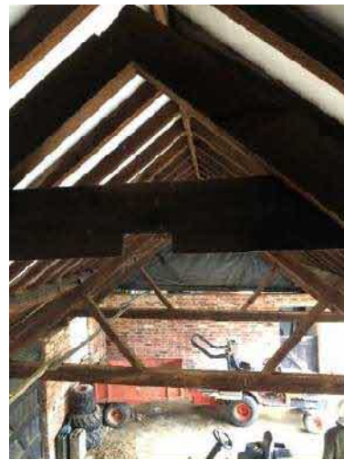
Figure 16. Square-sawn timbers of roof.
