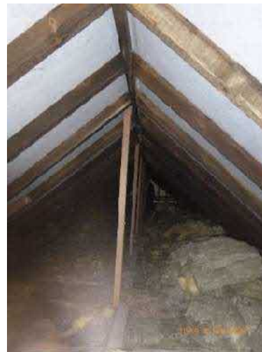
Figure 20. Eastern roof void.
