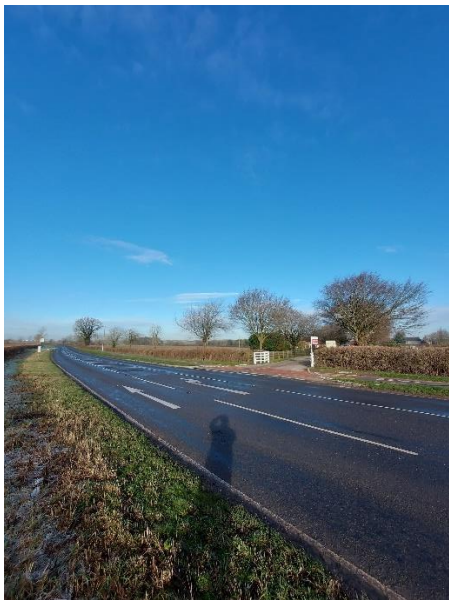
Photograph 3: Ghost island right turn lane at junction between A413 and Hanover Farm
