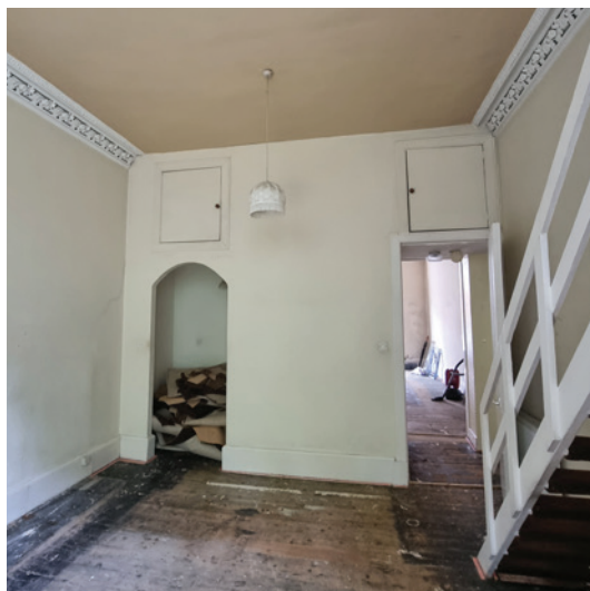
Existing partition to bedroom
