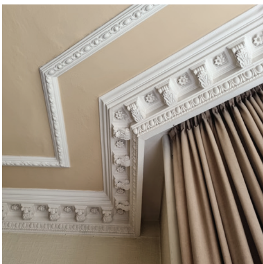
Living room cornice detail
