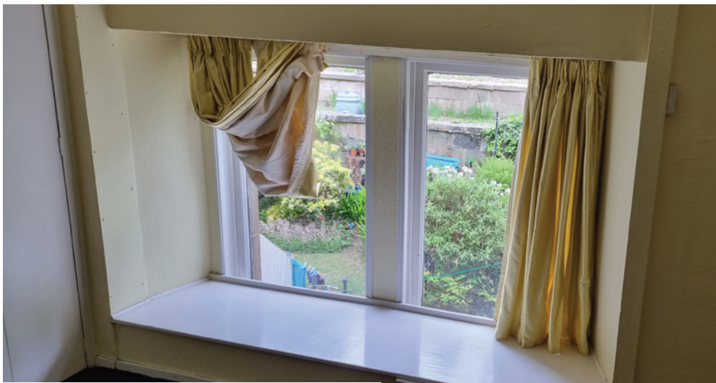
Divided window from Mezzanine
