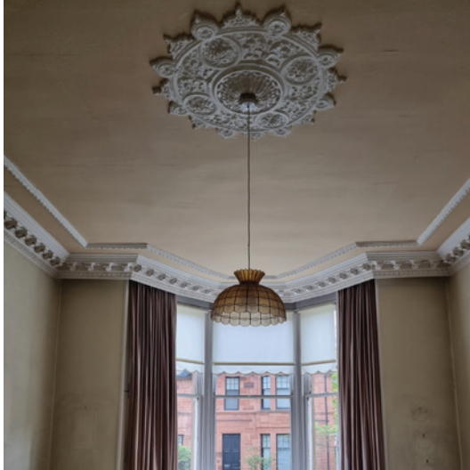
Living room features to be retained
