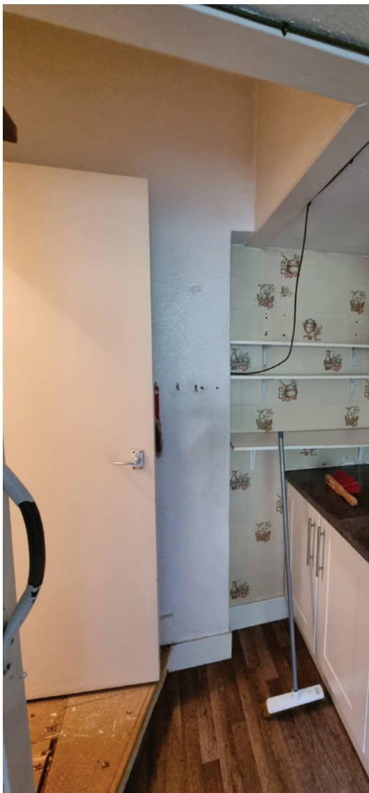
Kitchen showing step and roof void
