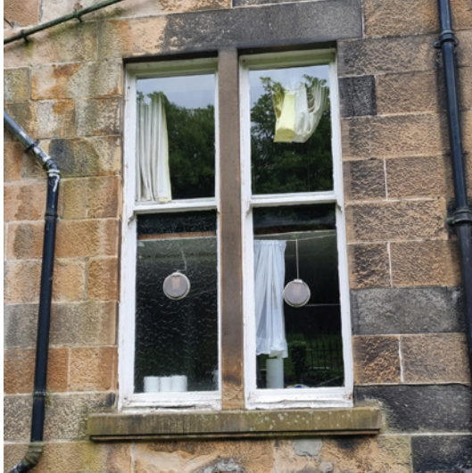
Divided window to rear room
