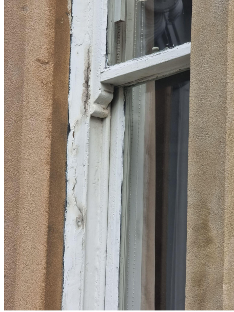
First photo shows missing sections of mastic and the casement bottom rail and sill are warped due to water damage. The second photo again shows broken mastic and signs of rotting within the casement.
