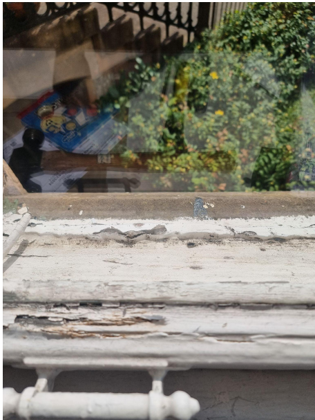
Photos show rotting bottom rail and sills to the windows.
