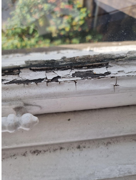
Paint has come away from the windows which is allowing water to enter the woodwork resulting in further rotting.
