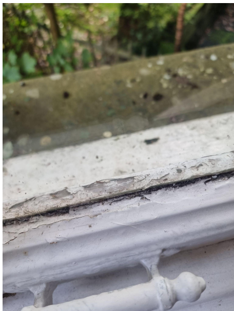
First photo shows the outside of the bottom rail is rotting and the second photo shows that the seals at the midrail have deteriorated and are allowing water to enter the woodwork and causing further rot and decay.
