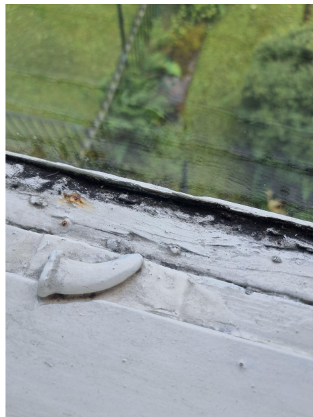
First photo shows the outside of the bottom rail is rotting and the second photo shows that the seals at the midrail have deteriorated and are allowing water to enter the woodwork and causing further rot and decay.
