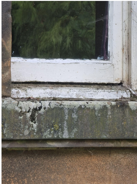
First photo shows a large gap between the bottom rail of the window and the sill which is allowing wind and water to enter the property. Both photos also show that the sills are rotting and deteriorating in sections.
