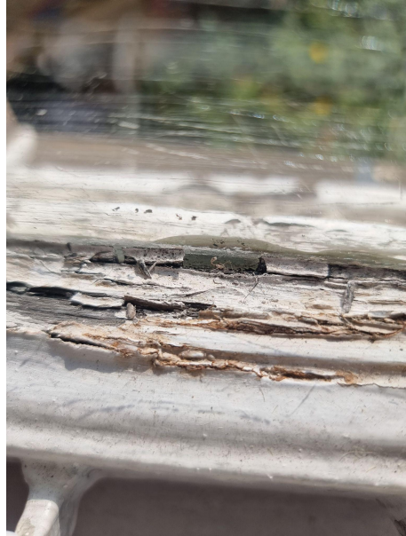
Photos show rotting bottom rails and broken seals.
