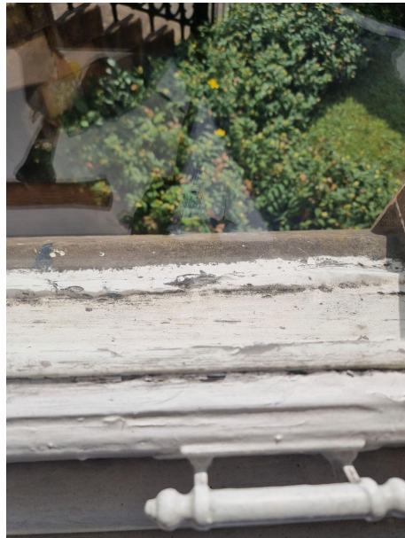
Photos show rotting bottom rail and sills to the windows.
