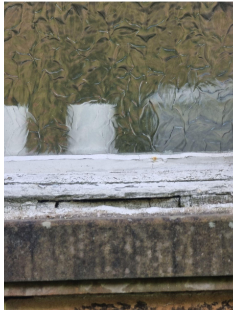
First photo shows a large gap between the bottom rail of the window and the sill which is allowing wind and water to enter the property. Both photos also show that the sills are rotting and deteriorating in sections.
