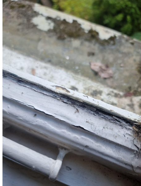
Photos show that the sashes and seals around the panes have failed, allowing water to enter the woodwork and causing rot and decay.
