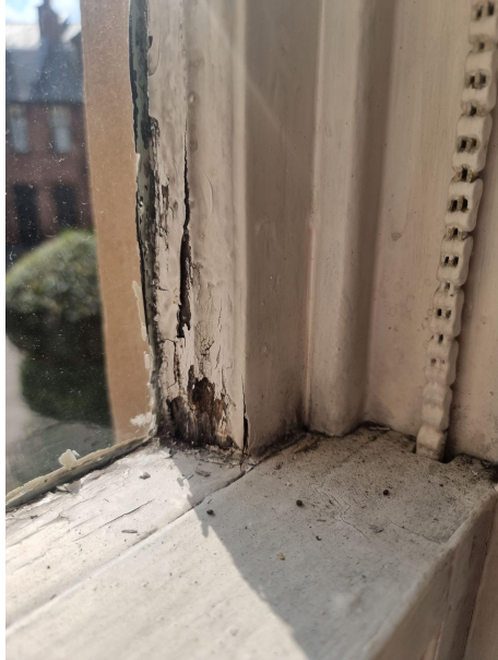
Photos show that the sashes and seals around the panes have failed, allowing water to enter the woodwork and causing rot and decay.
