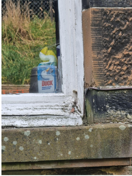
First photo shows missing sections of mastic and the casement bottom rail and sill are warped due to water damage. The second photo again shows broken mastic and signs of rotting within the casement.
