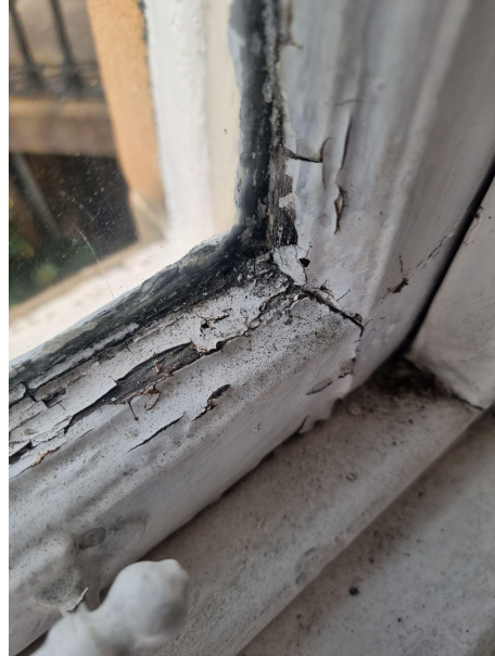
Paint has come away from the windows which is allowing water to enter the woodwork resulting in further rotting.
