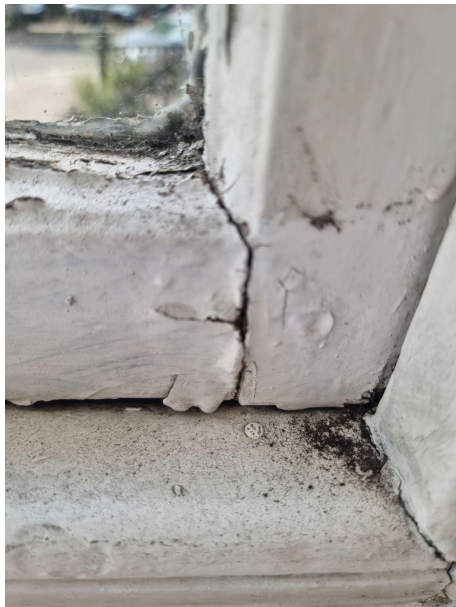
Photos show that the timber joints are failing and the sash woodwork is rotting.
