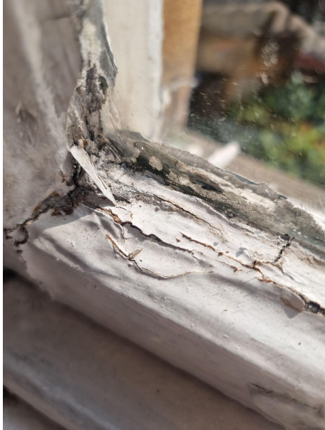
Photos show rotting bottom rails and broken seals.
