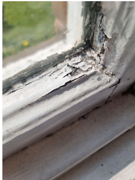
Photos show that the timber joints are failing and the sash woodwork is rotting.
