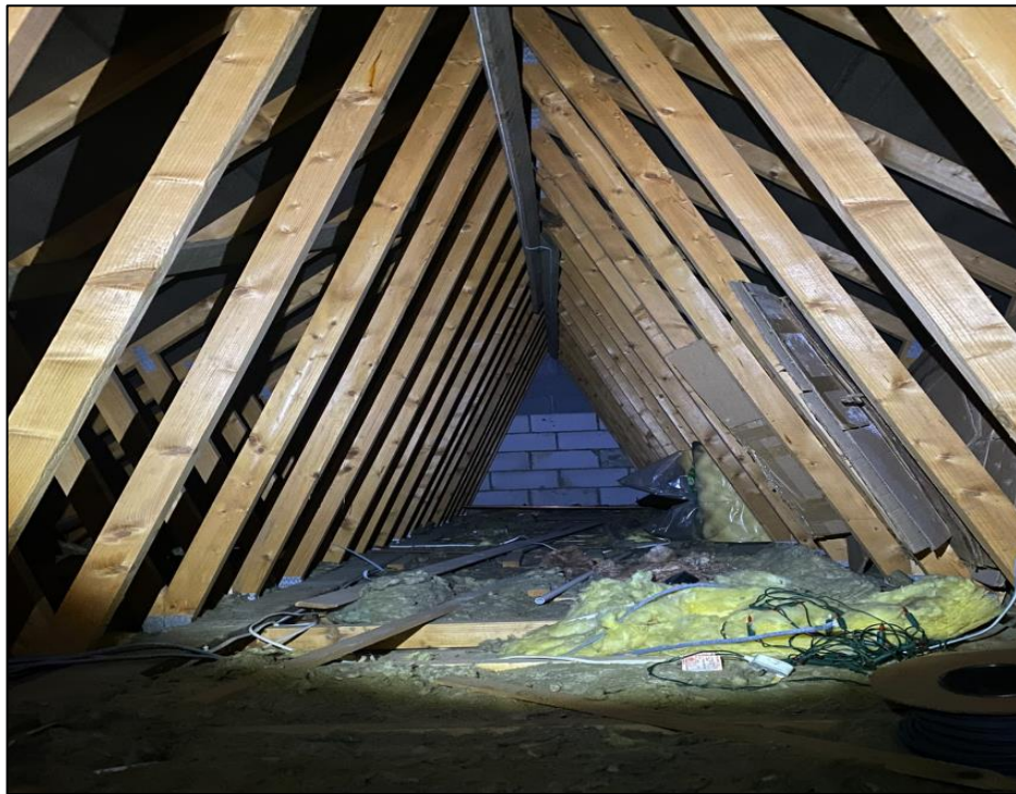
Plate 4: An internal photograph of the first accessible roof.
