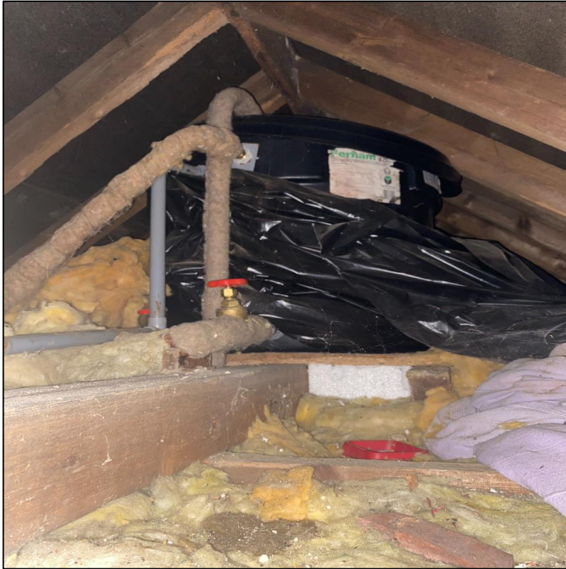
Plate 7: Internal photograph of the third accessible roof
