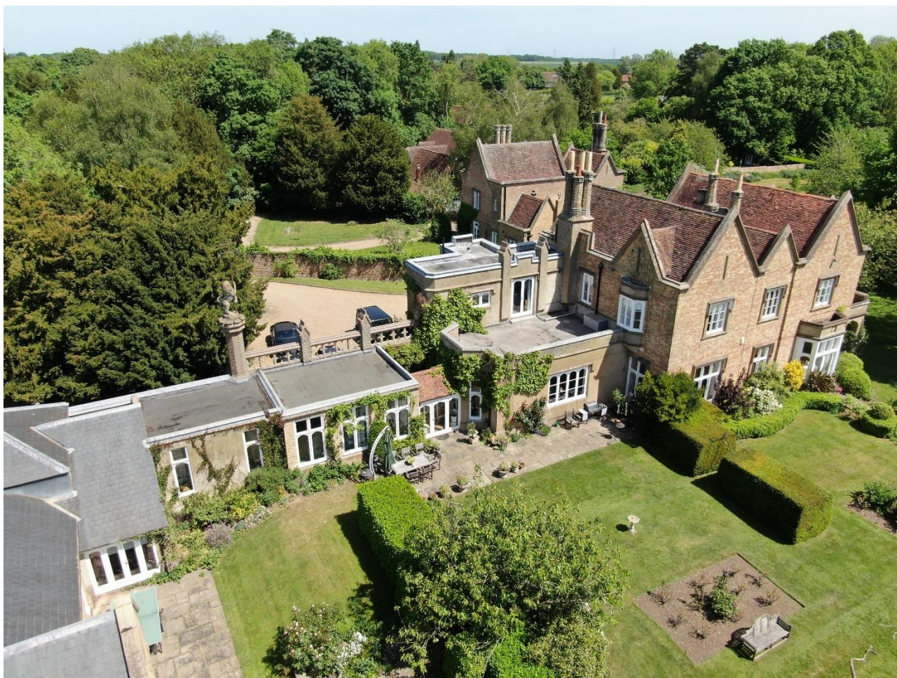
Photo 1: An aerial view of Hunsdonbury, from the SW, with the Gate House seen in the distance behind.
