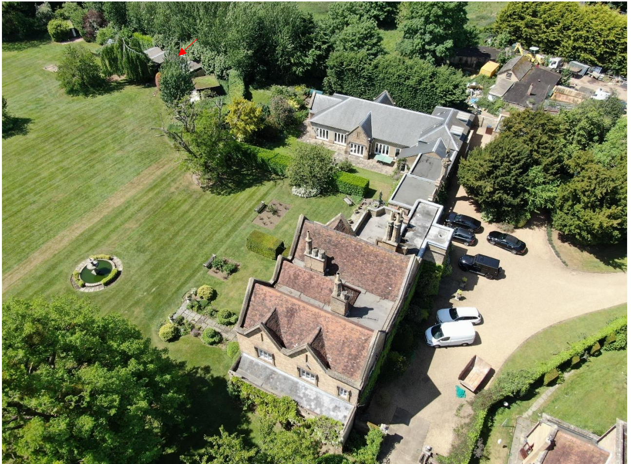
Photo 4: An aerial view of Hunsdonbury in its context, from the NE, with the red arrow showing the stables on the application site.
