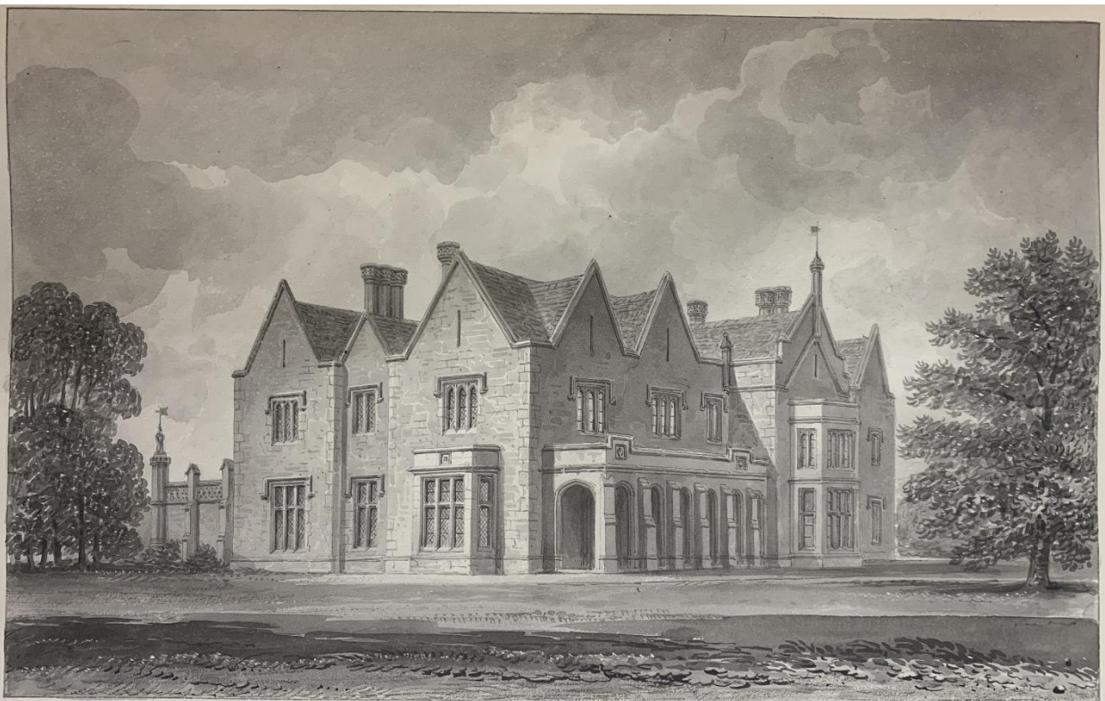
South East View of the Parsonage House at Hunsdon, Hertfordshire.
