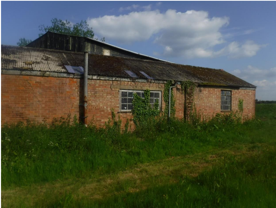
Barn in north west corner.
