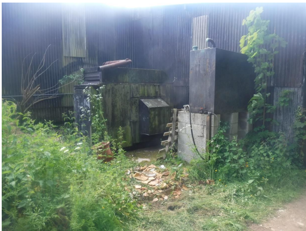
Above ground storage tank and grain dryer unit.
