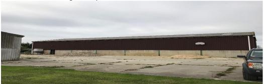
6.2 The building consists of a steel portal with steel sheeting rails with steel and timber roof structure. The timbers are in good condition and adequate to take normal residential loads associated with all commonly used roofing materials.
