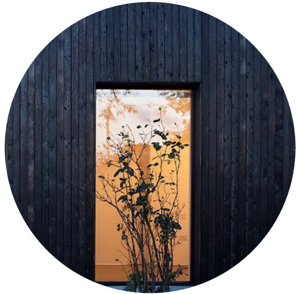
Timber-framed glazing - no mullions, allowing it to read as a distinctively new feature
