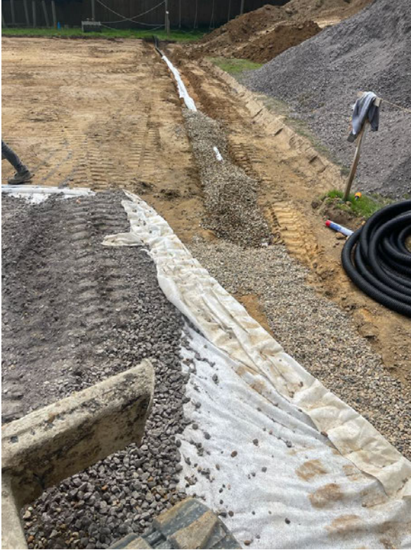
Plate 4. trench filled and geotextile at formation with MOT Type 3 being spread
