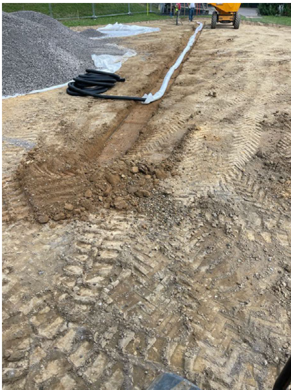
Plate 1. Formation dig and laying of sleeved pitch drain
