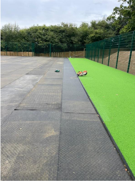
Plate 6. Shockpad installed and synthetic surface partially laid
