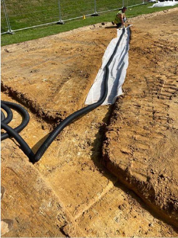
Plate 2. Pitch drainage pipework in trench
