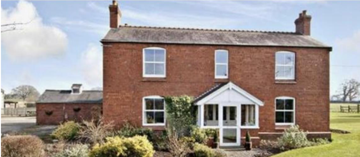
Figure 2 – The existing main farmhouse (Lodge Farm)
