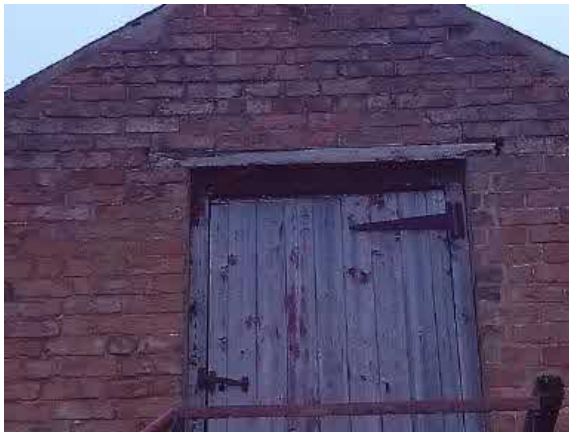
Photograph 3: Gap under door on B5 with bats recorded emerging and re-entering
