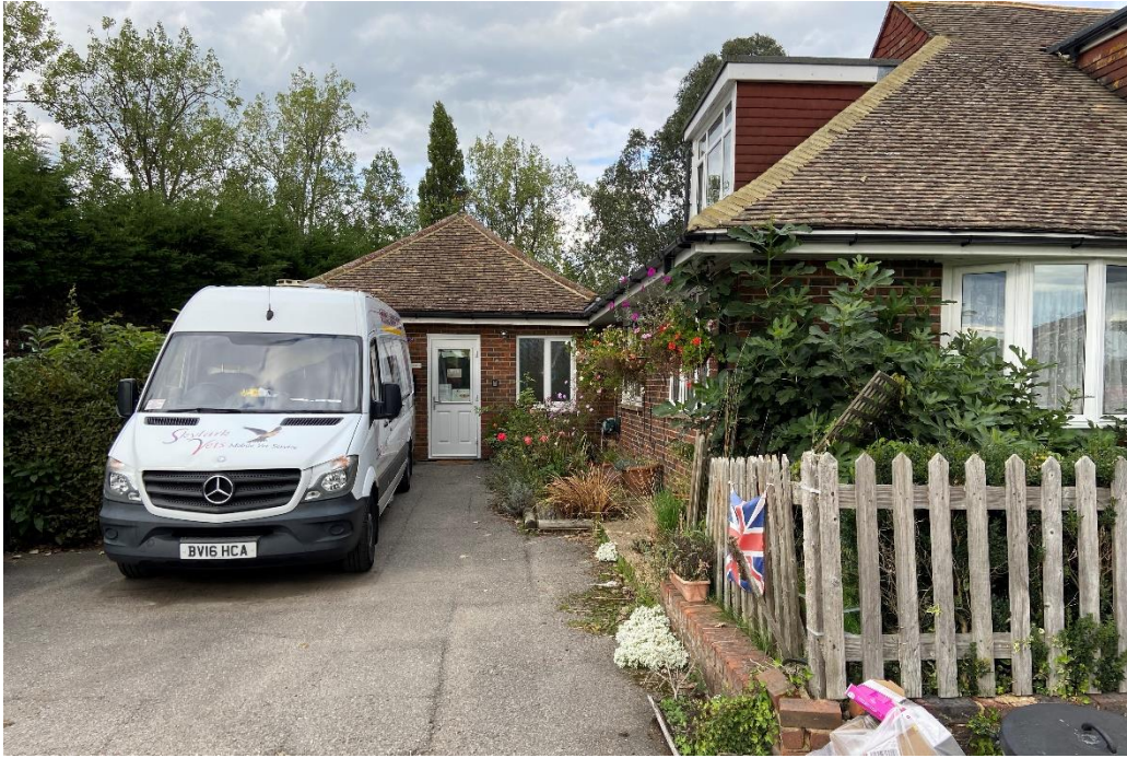
Figure 3: Picture showing the bungalow to the right-hand side and the Vets practice (converted garage) behind the van.
