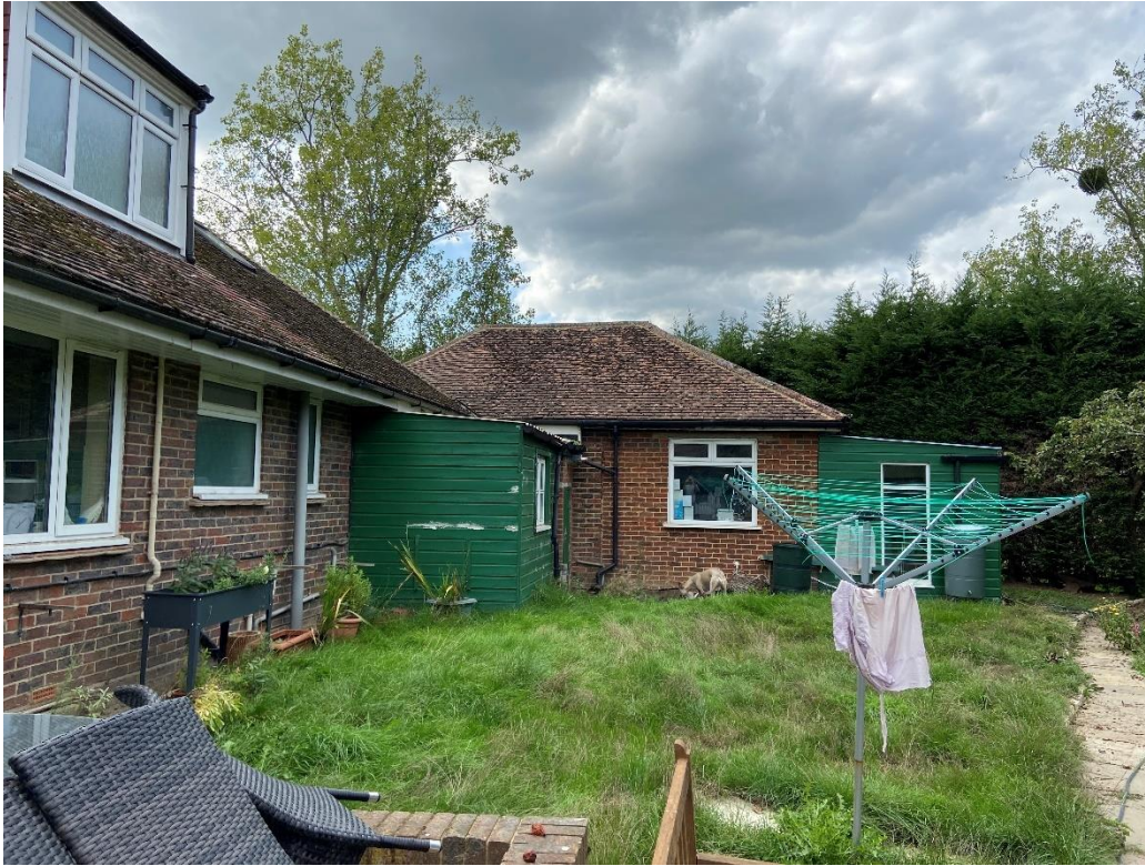
Figure 4: Showing the rear of the vets practice from the residential garden.
