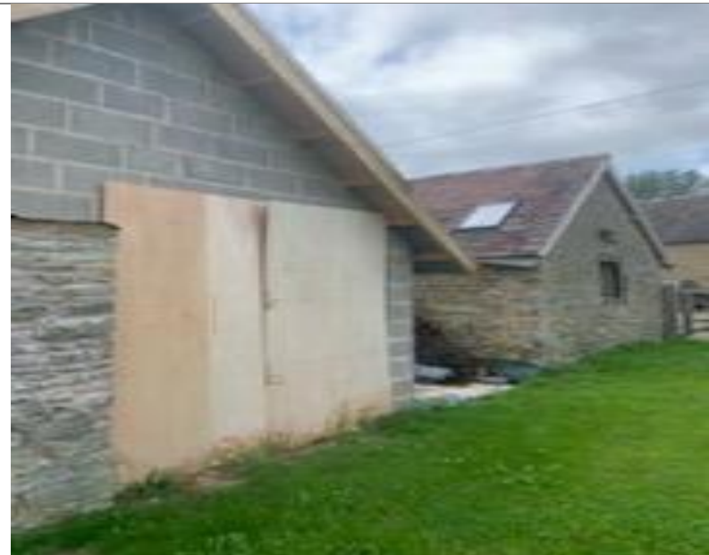
GABLE END OF RECENT GARAGE AND STABLE BLOCK BEYOND
