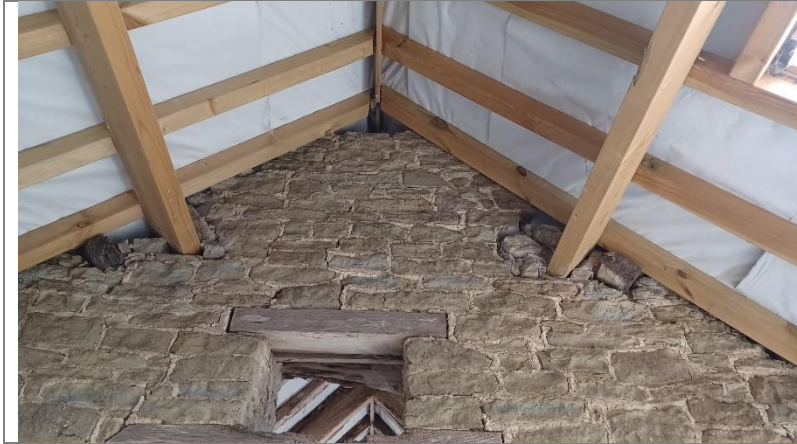
INTERNAL OF STABLE BLOCK SHOWING REPAIRED ROOF STRUCTURE
