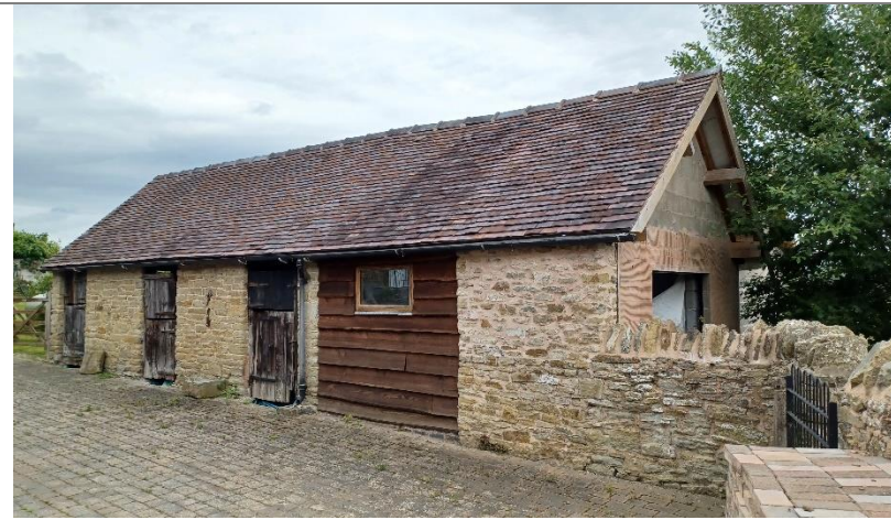
FORMER STABLE BLOCK
